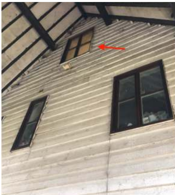
Existing, modern window for replacement
