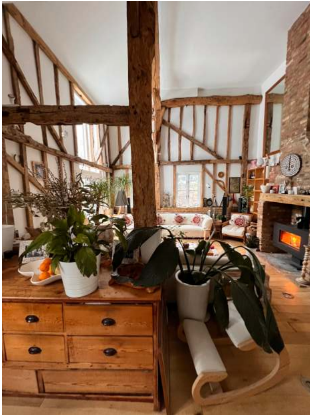
Exposure of the original timber posts and beams is a positive internal feature, providing a constant and evocative reminder of the building's agricultural origins and architectural significance
