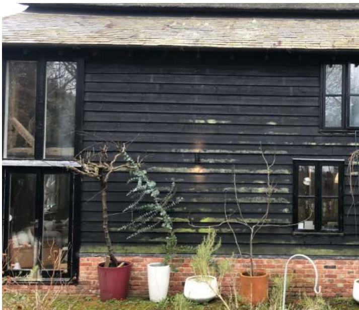
Ambient downlight - illuminated
