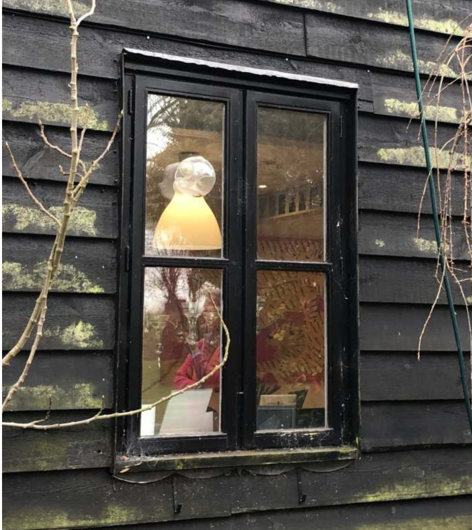
Close-up image of window style
