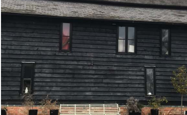
Arrangement of windows across the front elevation
