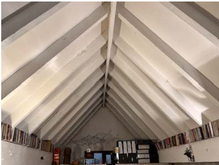
Internal view of the 1980s roof
