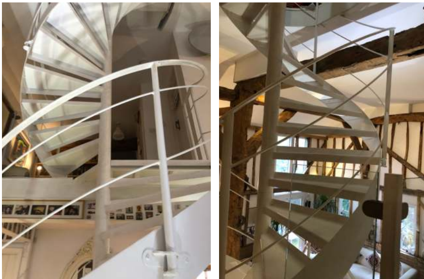
Interior stair has a simple, functional character that relates well to the agricultural style of the converted barn. Its compact form and open tread preserves much of the building's original open plan form and long sight lines
