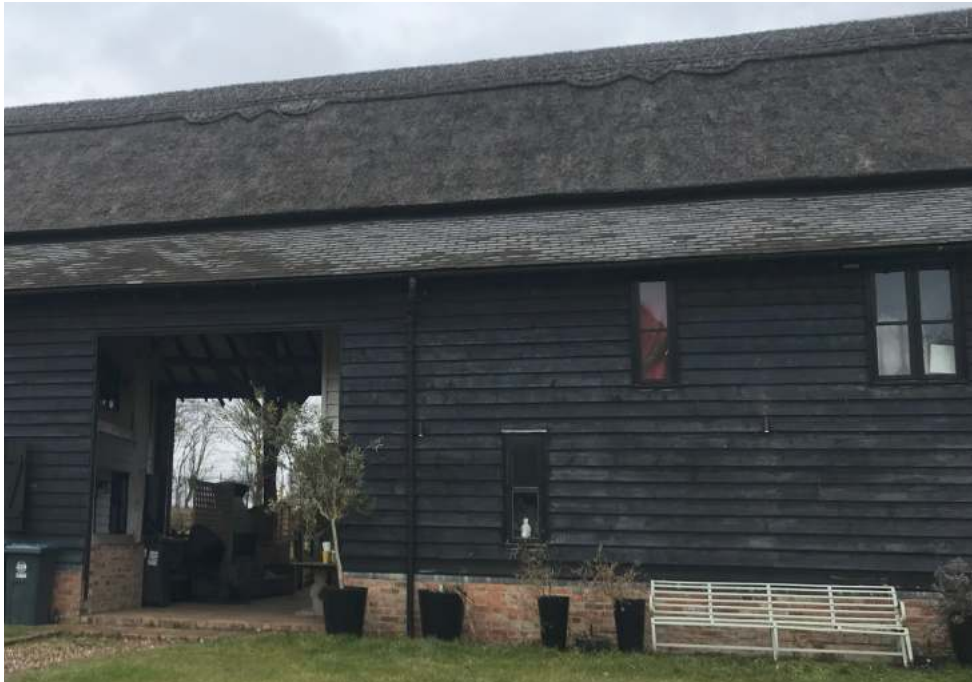
Dark-stained weatherboarding atop a brick plinth
