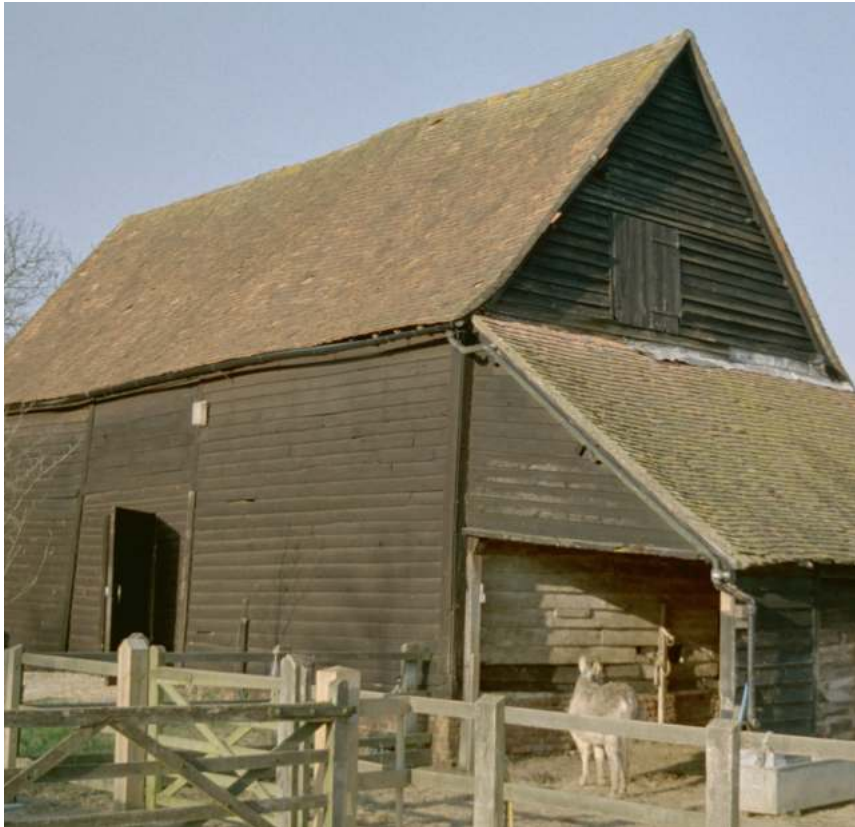
Example of a hay door located in the upper gable of a traditional rural barn
