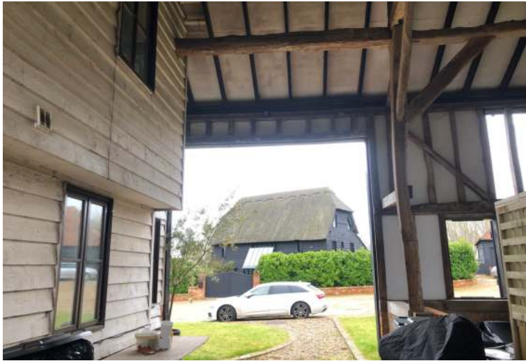
View of the neighbouring, curtilage-listed barn conversion (The Garden House) from the host property
