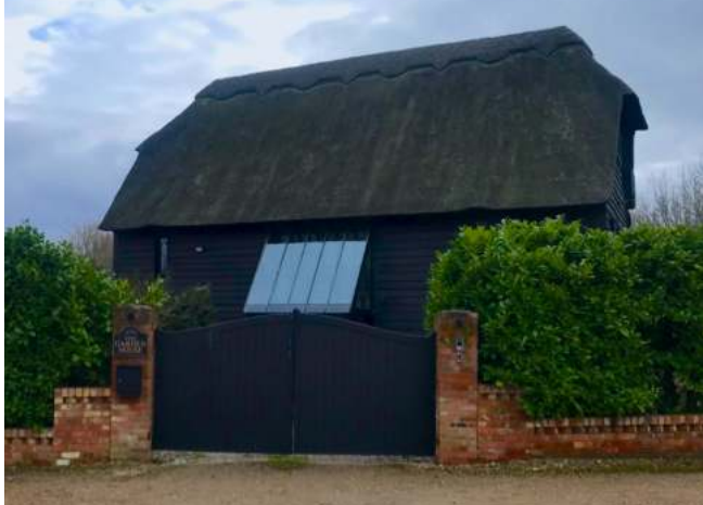
Recent photograph of neighbouring barn conversion “The Garden House” - although not individually listed, the building possesses clear heritage value and is likely to be considered curtilage listed
