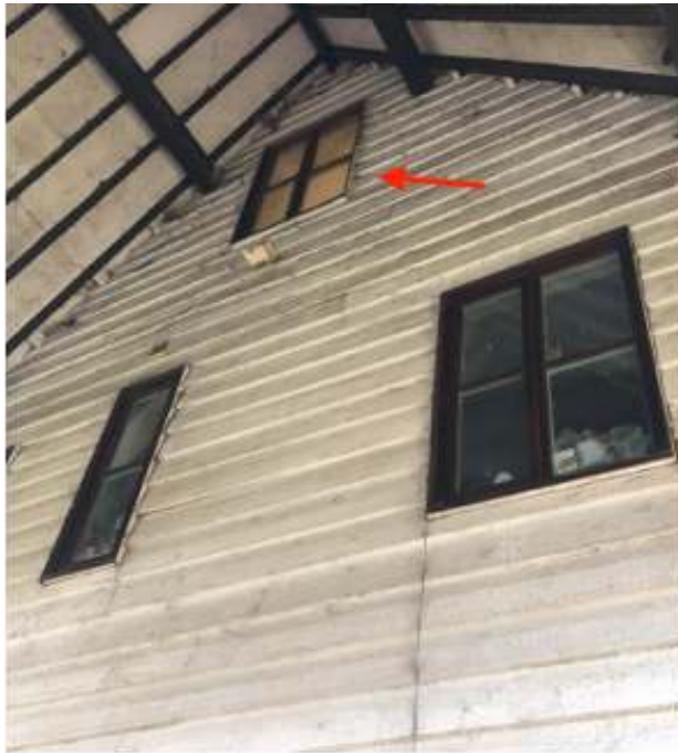
Existing, modern window for replacement
