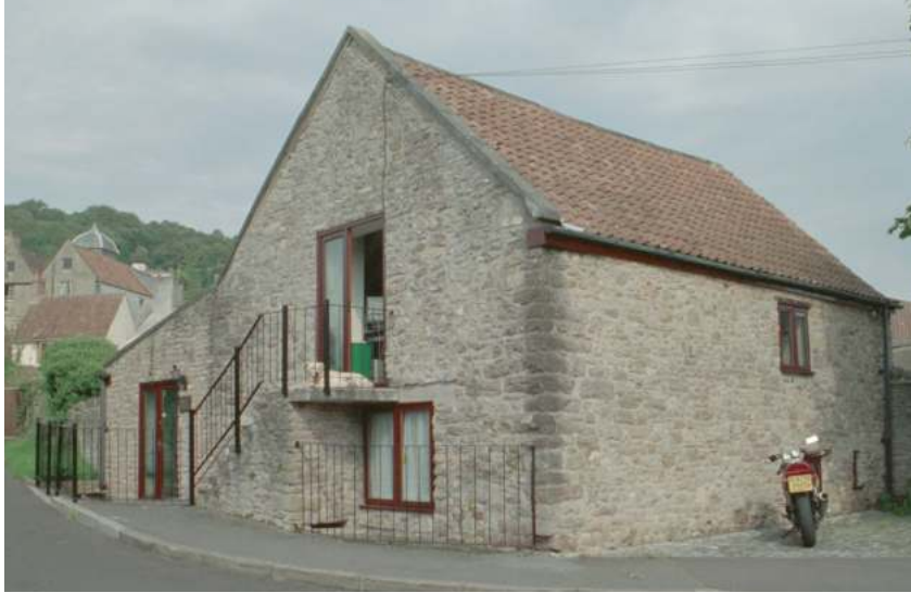
Example of a historic stair attached to a GII C15 barn in Somerset - Historic England archives (reference IOE01/03046/28). The stair itself is built-in but significantly makes use of simplistic, dark metal railings
