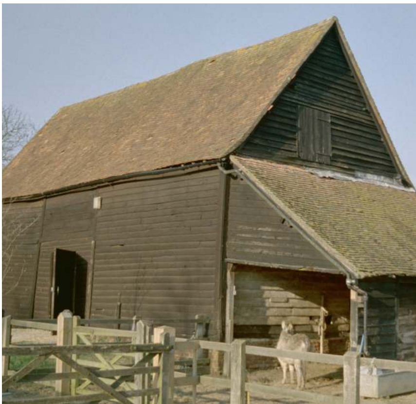
Example of a hay door located in the upper gable of a traditional rural barn
