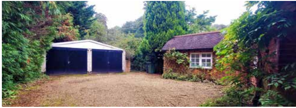
Fig. 33 - Existing garage within site context
