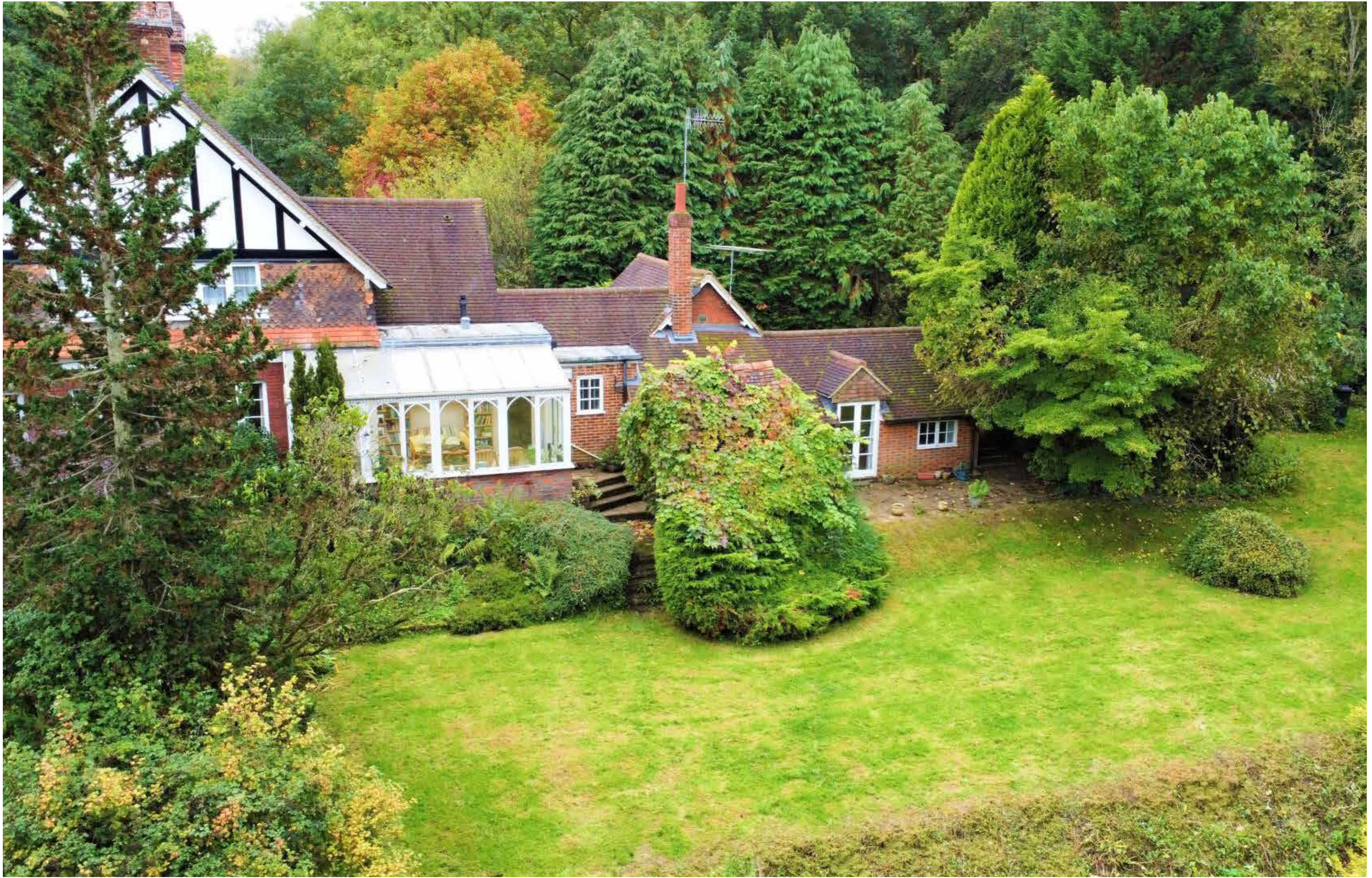
Fig. 02 - Aerial view of site
