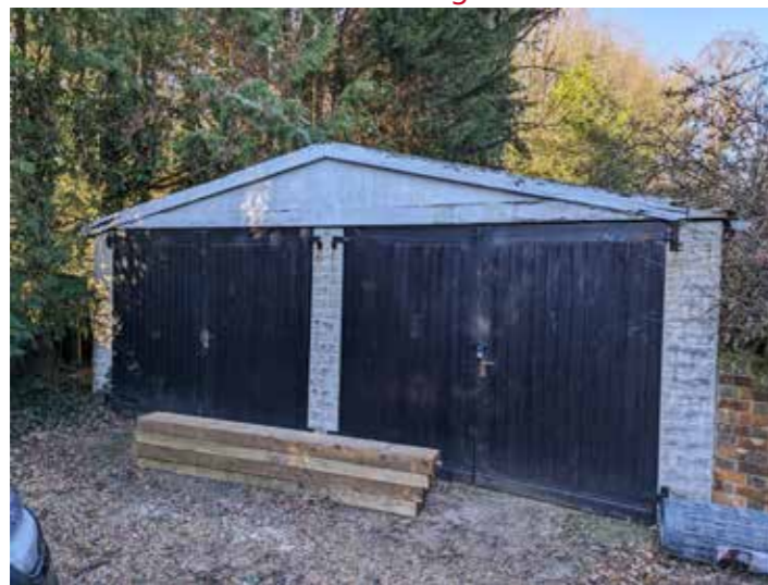
Fig. 45- Front view of existing garage
