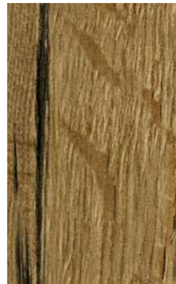
Oak frame for flat roof rear dormer
