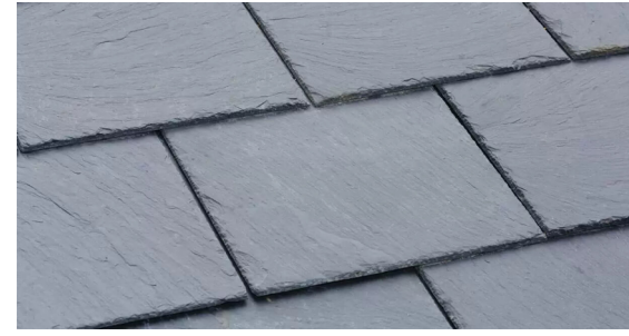
TRADITIONAL SLATE ROOFING
