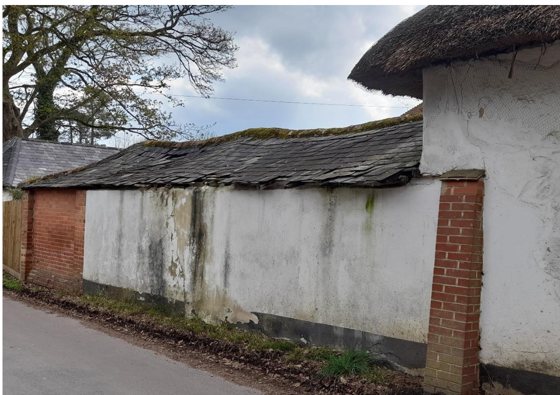
Fig. 27: The rear, roadside elevation of the single-storey eastern range.
