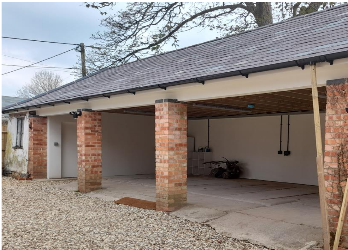
Fig. 30: The west elevation of the unlisted converted building at the eastern side of the courtyard.
