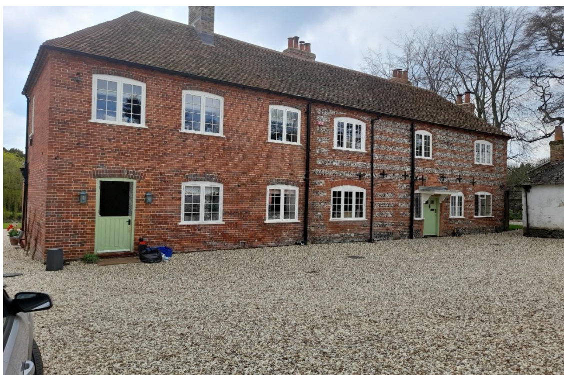
Fig. 6: The north, rear elevation of Bec House, looking south-west.
