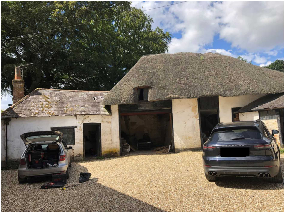
General View of Building Range - Front Elevation
