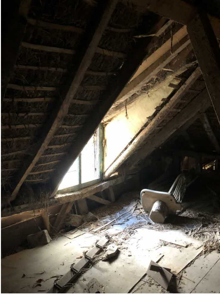
View of Internal Roof Structure Looking at Dormer Window
