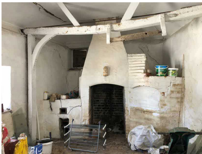
View of Bothy End Wall, Ovens and Cross Frame
