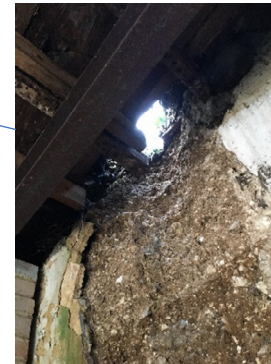
Due to failed thatch, water ingress has caused damage to cobb wall and timbers
