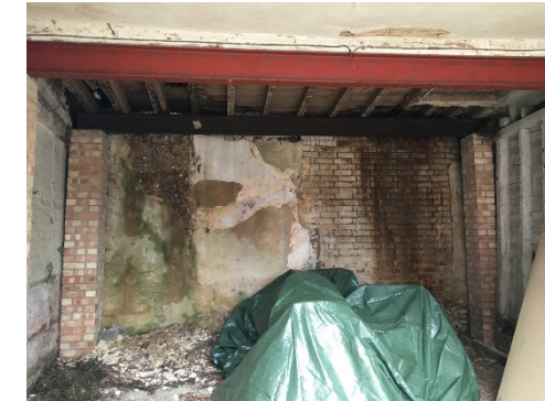
Due to failed thatch, water ingress has caused damage to cobb wall and timbers
