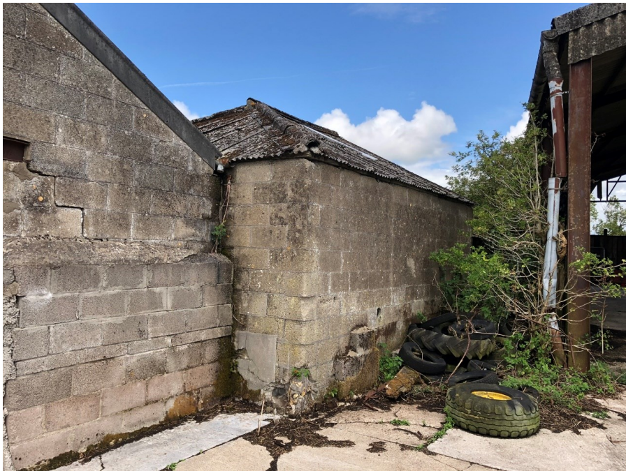
Junction with Farm Building at N-E Corner
