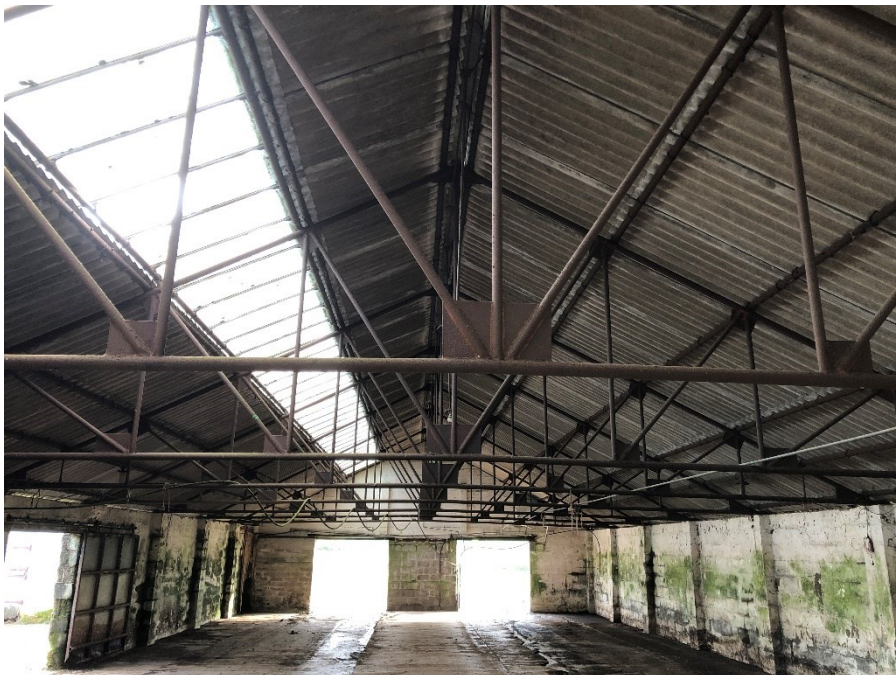
Interior Looking East
