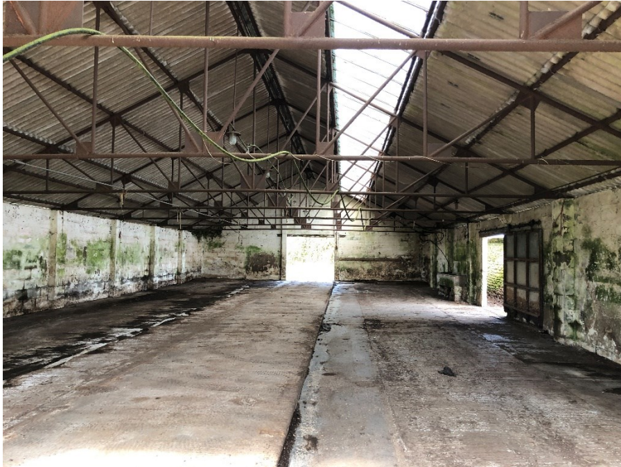
Interior Looking West
