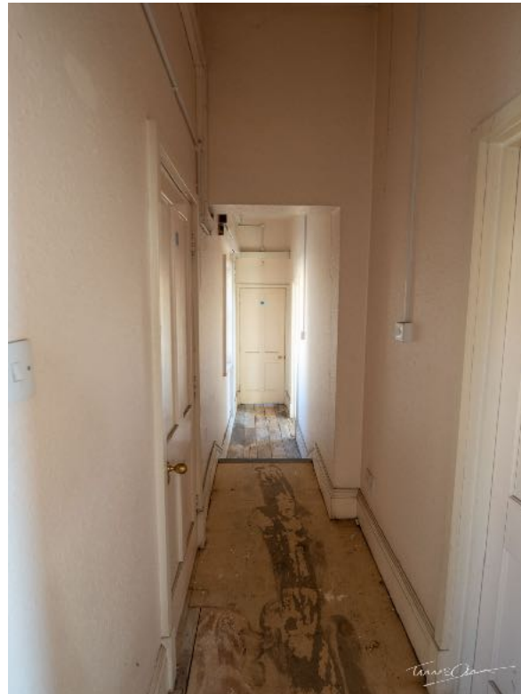
Existing corridor to rear range retained
