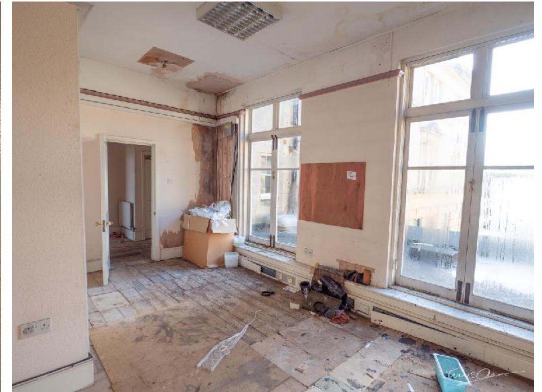
Rear of proposed flat 2 showing door opening to be blocked
