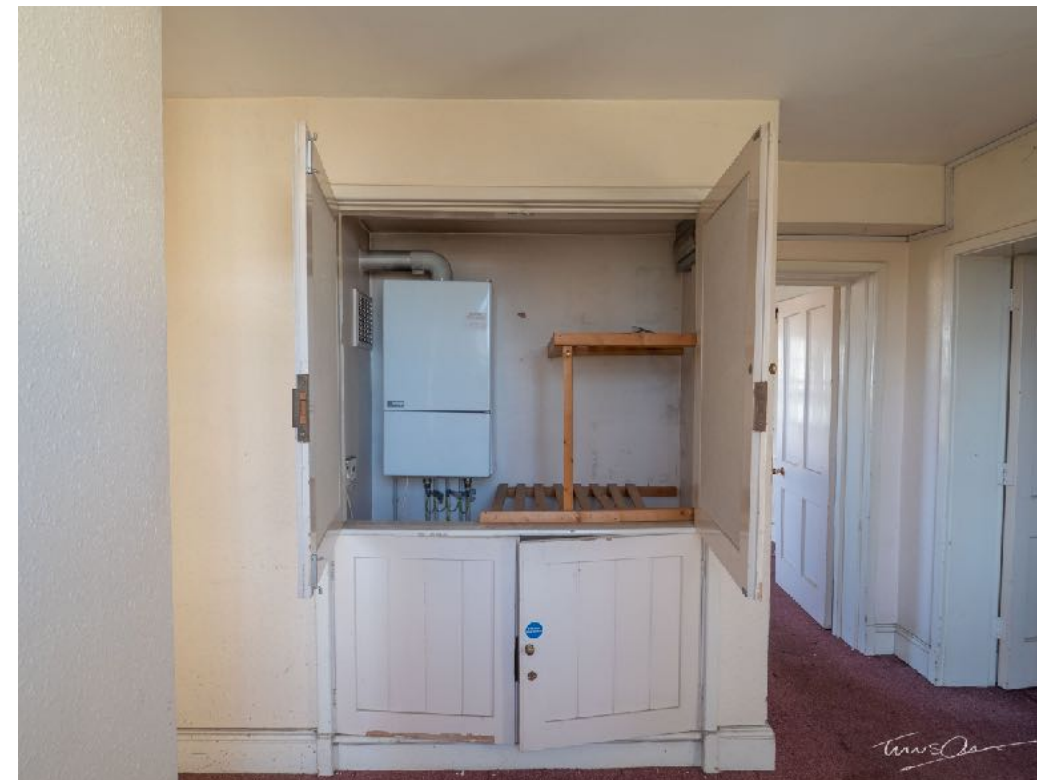
Boiler cupboard to be removed forming new bathroom
