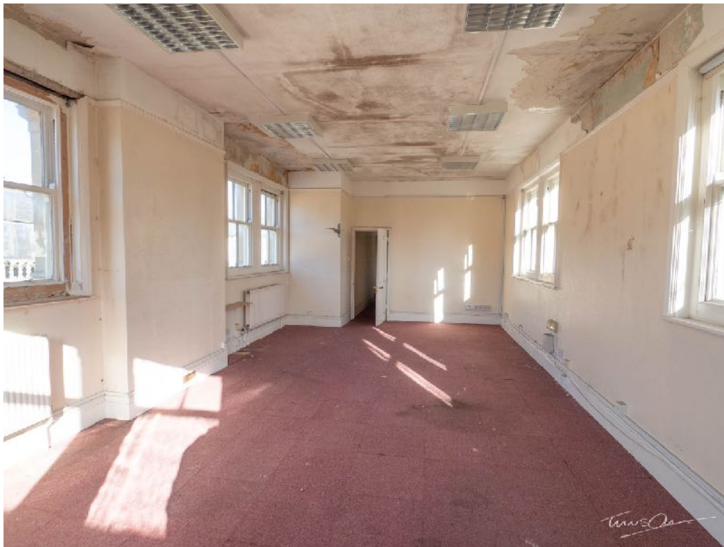
Rear range 2nd flr showing proposed area of new staircase
