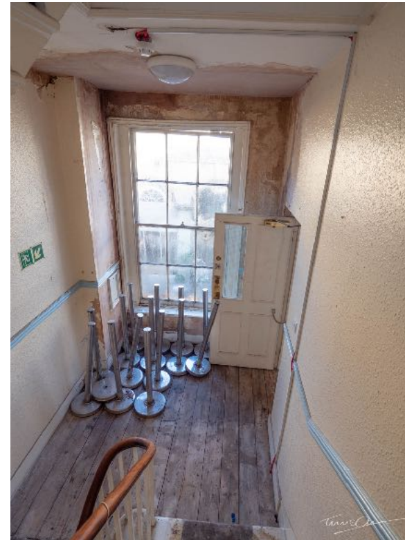
Staircase where lightweight lobby to be installed
