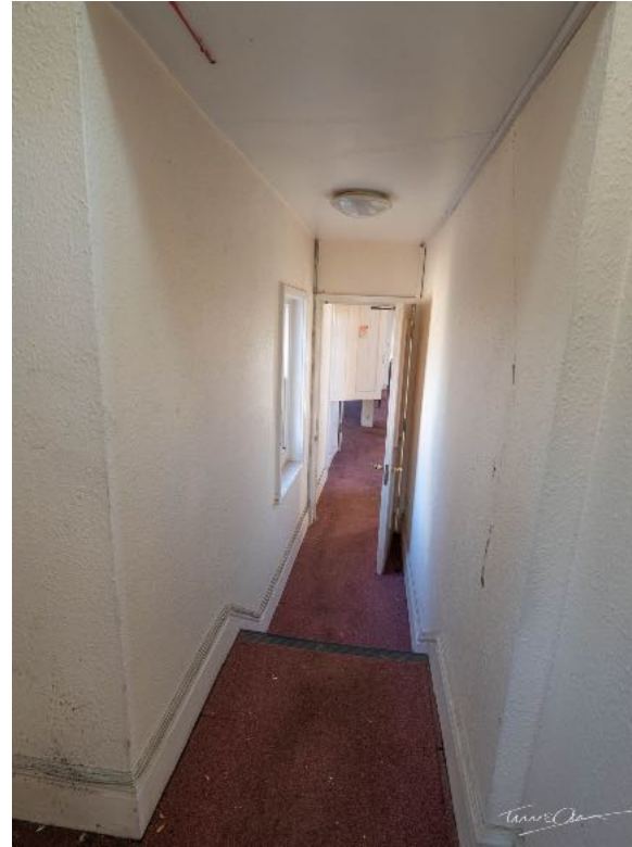
second floor partition rhs to be removed
