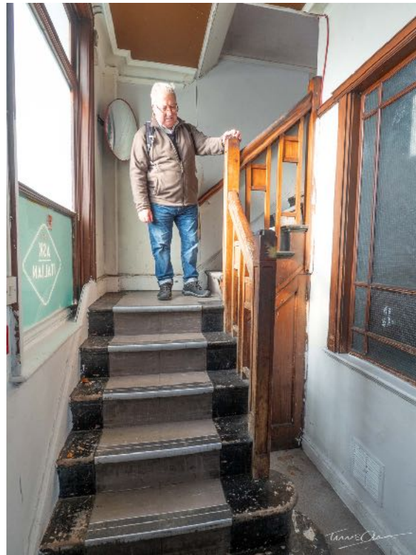
Existing entrance stair to be retained
