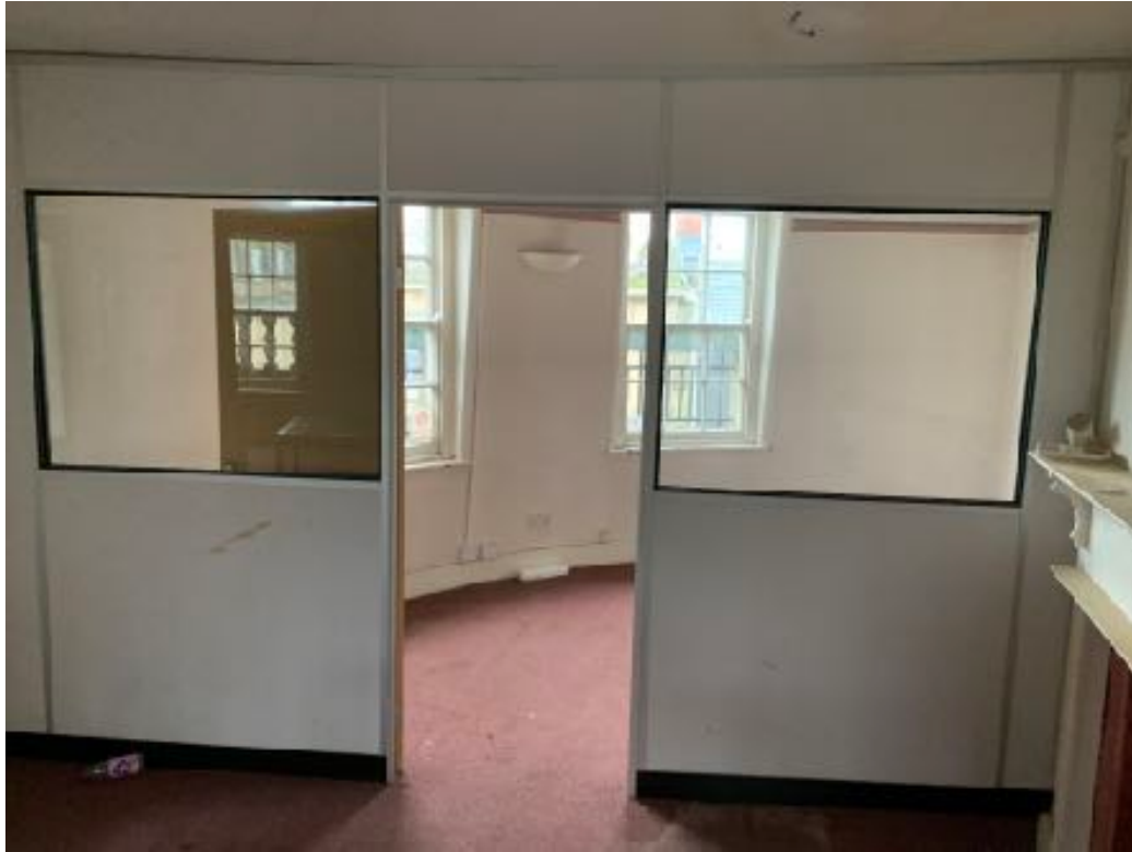
Partition to be removed on second floor
