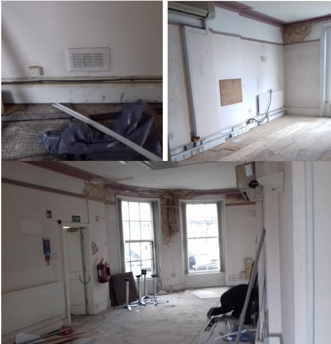
Figure 8.3 Air brick/air conditioner on first floor, second floor fireplace not shown
