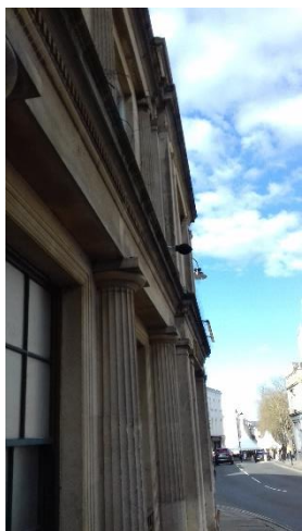
Long term monitoring position UN-01 (east façade)
