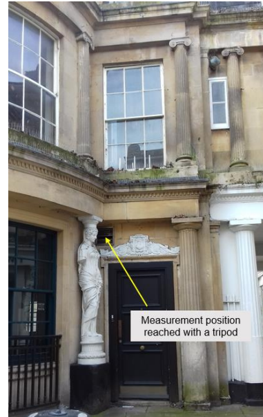
Short term monitoring position AT-03 (west façade vent.)
