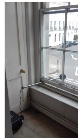
Long term monitoring position UN-01 (east façade)
