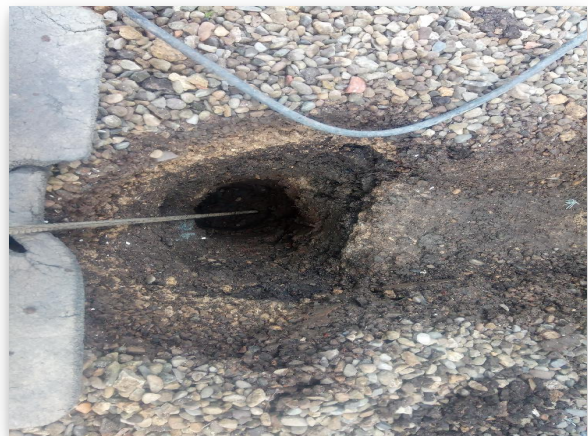
Fig 1.2: Trial Hole 1 Footing
