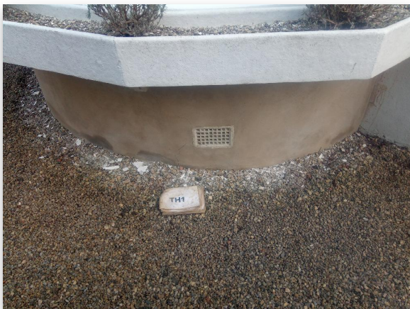
Fig 1.1: Trial Hole 1 Location
