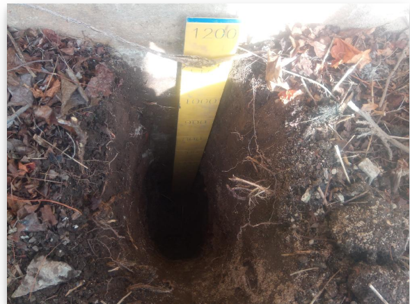
Fig 3.2: Trial Hole 3 Footing
