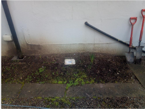
Fig 2.1: Trial Hole 2 Location
