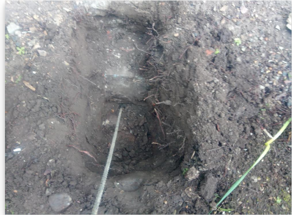
Fig 2.2: Trial Hole 2 Footing
