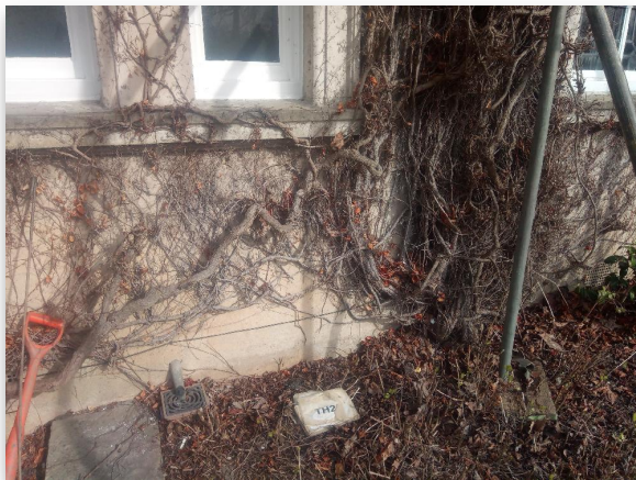
Fig 3.1: Trial Hole 3 Location
