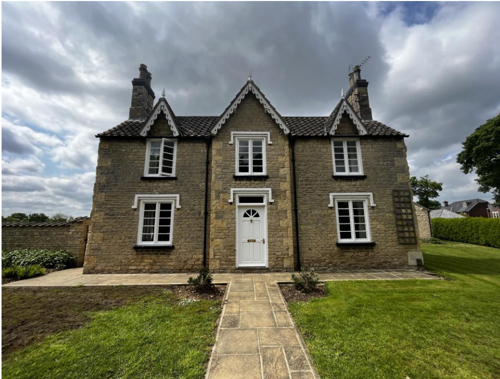
Figure 2- MANOR FARM PRIMARY ELEVATION FACING CHURCH HILL ROAD
