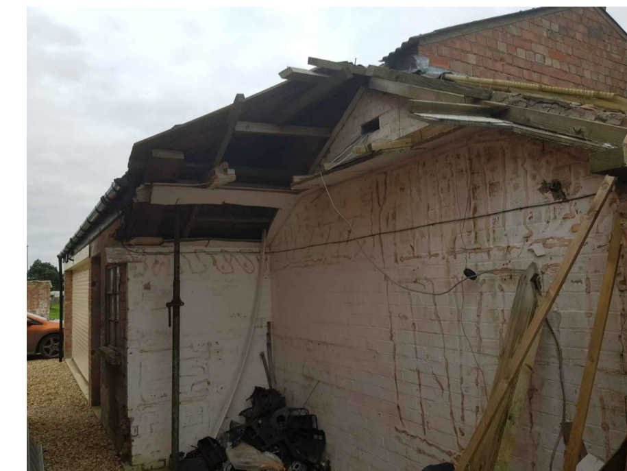
photo partially demolished area
