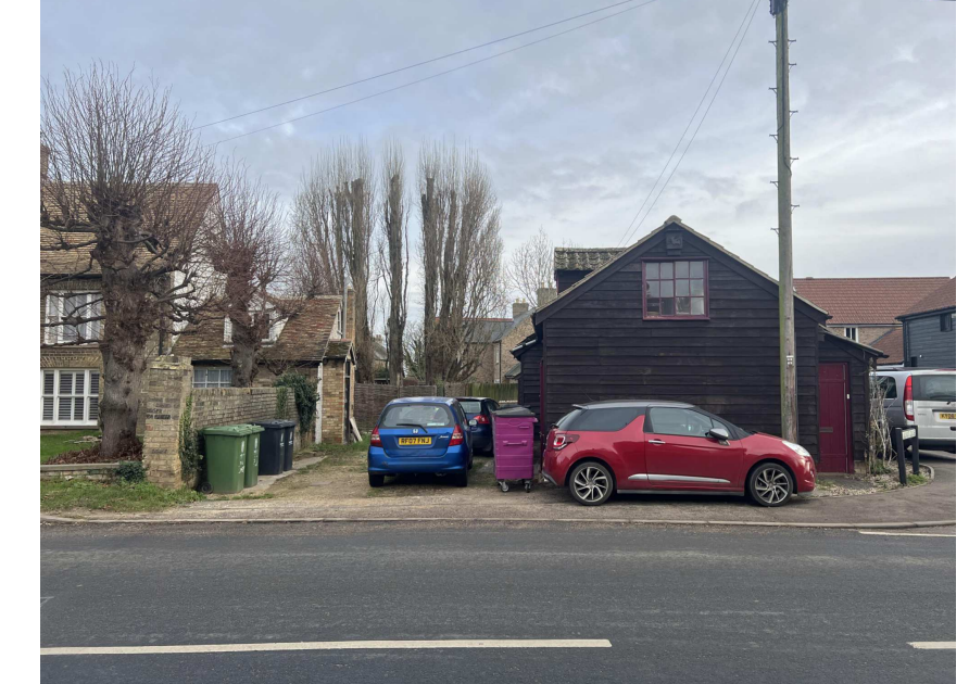
EXISTING PARKING AREA ACCESS
