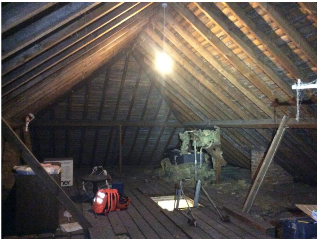
Photograph 13. Showing the uncluttered internal loft void, lined with wooden sarking with rockwool and wooden boarding at ground-level.
