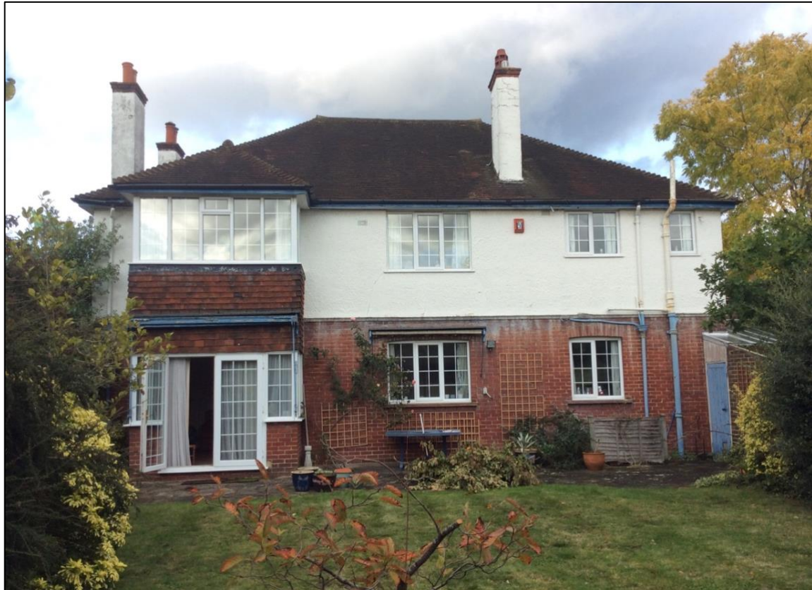
Photograph 3. Showing the rear (southern) aspect of the main residential dwelling, with associated paved area.
