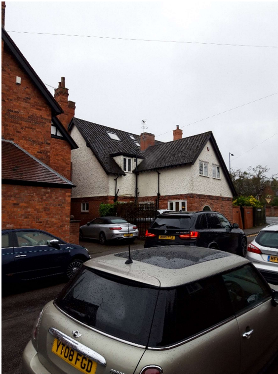
Photo of neighbouring house with rooflights to front elevation
