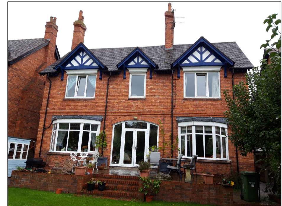
Photo of Rear Elevation
