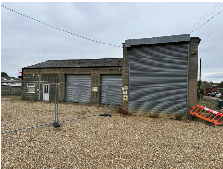
Photo of Site
