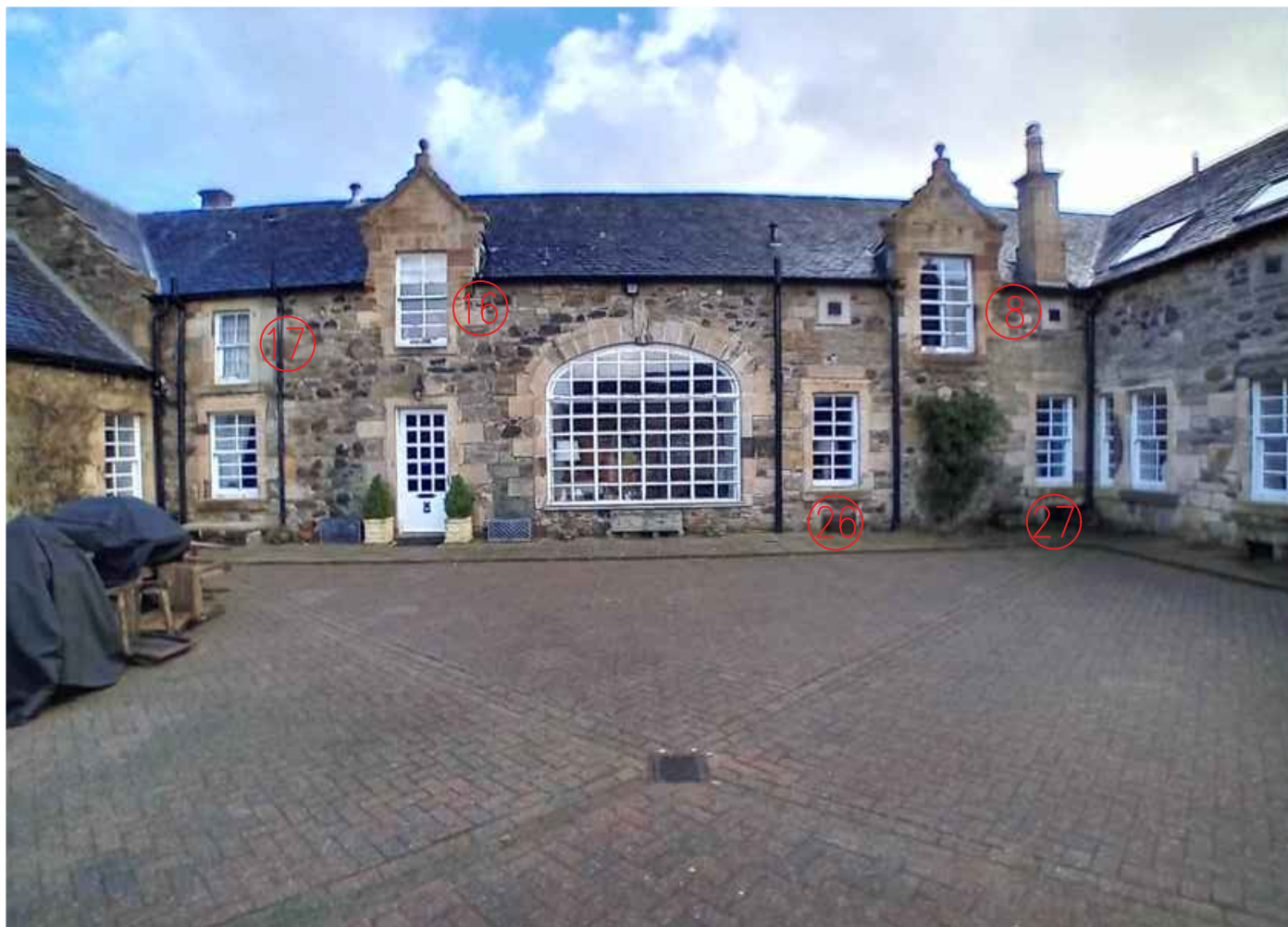
photo of (south west) elevation as existing viewed from courtyard. nts.
