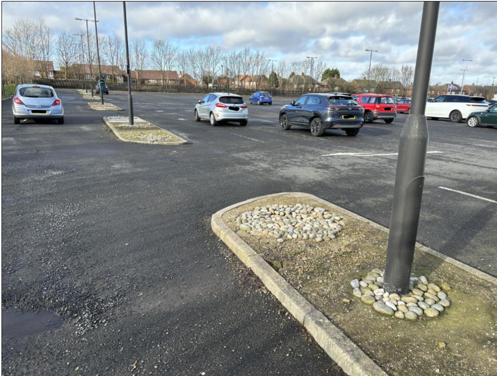
Image showing hardstanding (car parking) which is present throughout the proposed development site
