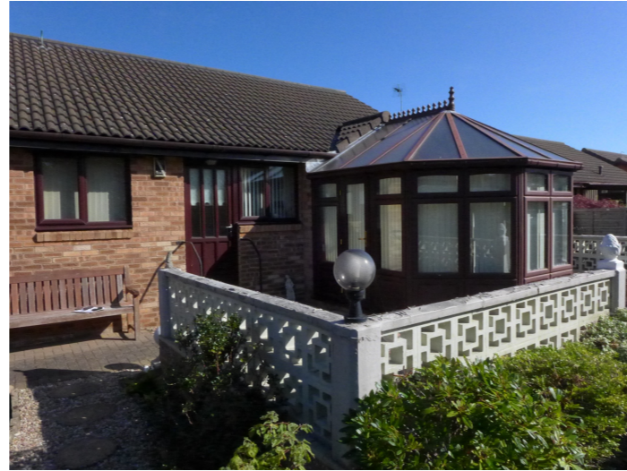
2. VIEW FROM REAR GARDEN LOOKING NORTH-EAST
