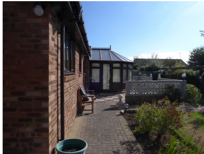
4. VIEW FROM REAR GARDEN LOOKING EAST
