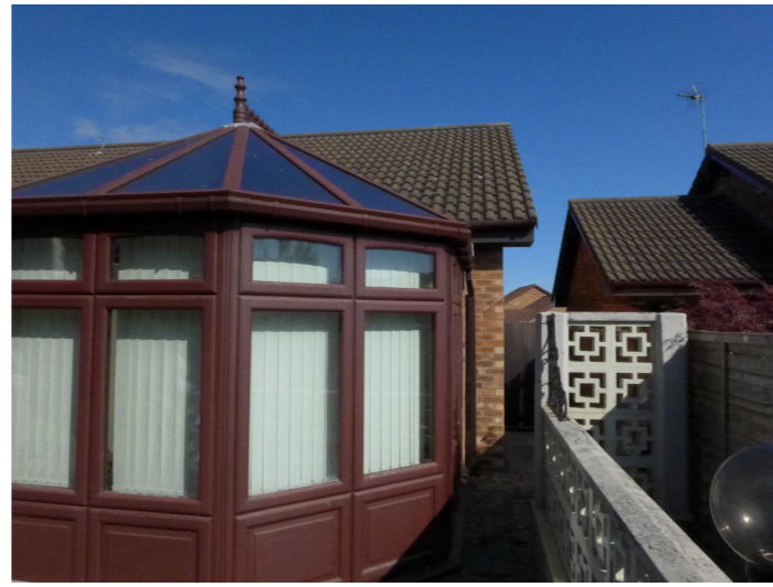
5. BOUNDARY WITH 32 LORD PRESIDENT ROAD VIEWED FROM REAR OF HOUSE
