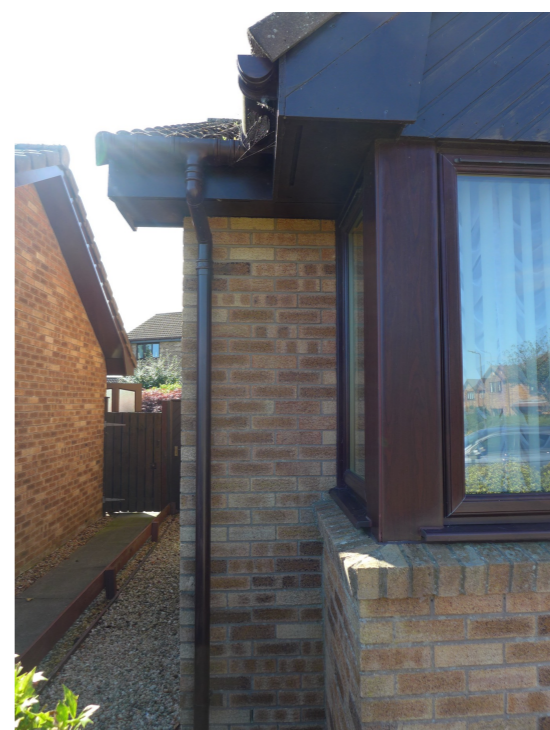
6. BOUNDARY WITH 32 LORD PRESIDENT ROAD VIEWED FROM FRONT OF HOUSE
