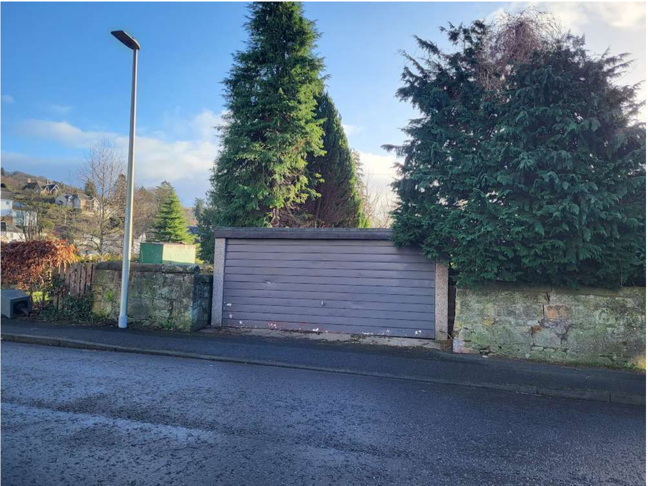
EXISTING VIEW WEST FROM GRAHAM STREET
