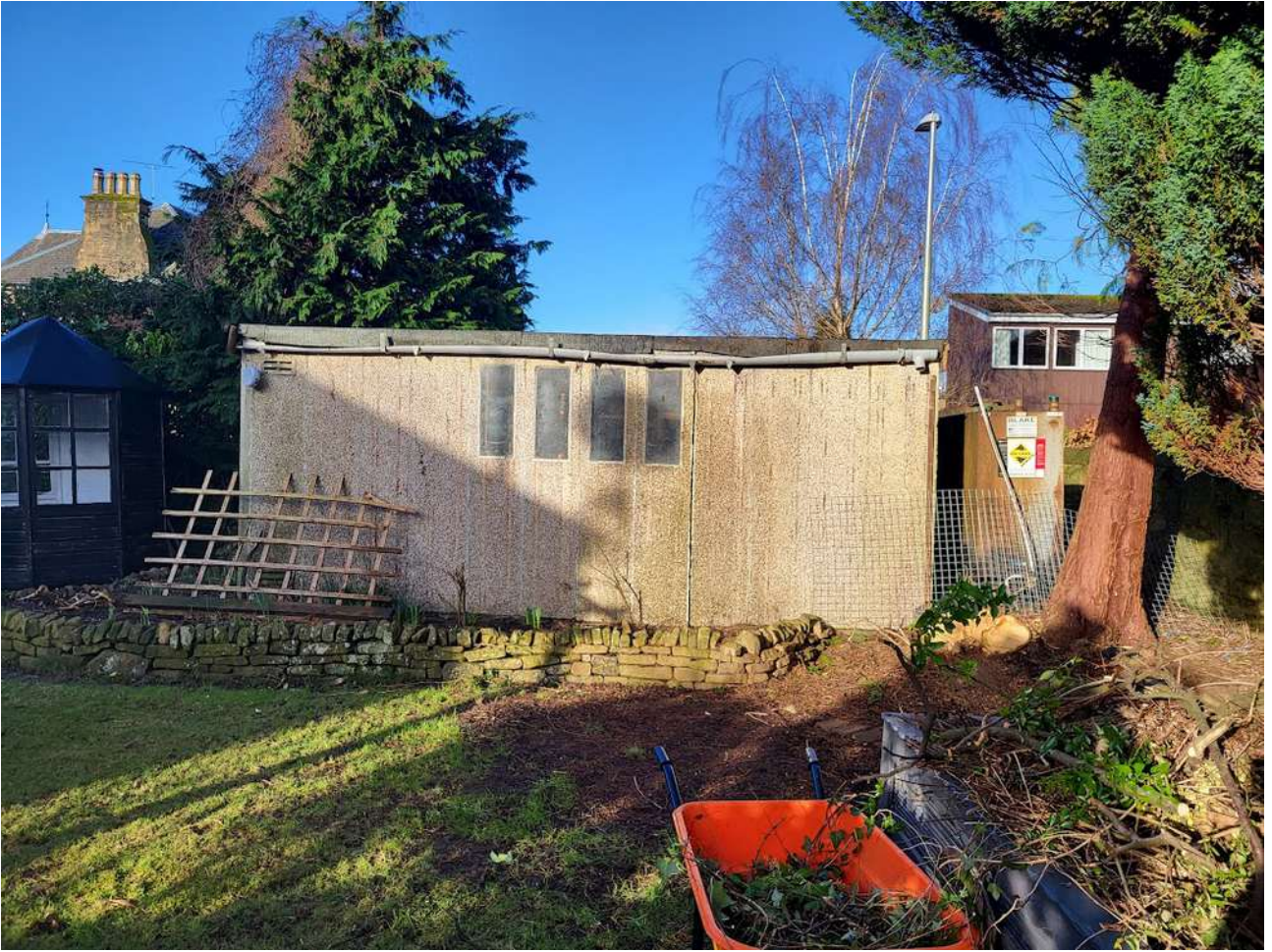
EXISTING VIEW EAST FROM GARDEN
