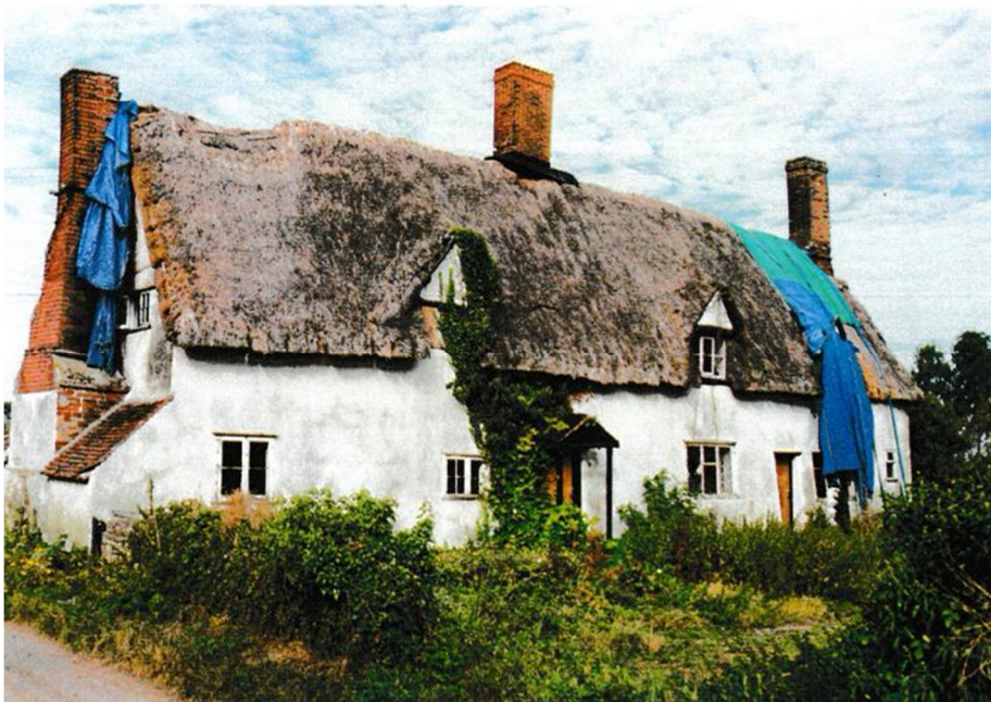
Figure 3. Historic photograph of Northeast (pedestrian entrance) elevation showing previous roof, dormers, windows, doorways and porch. The porch is now the position of a window and the door has been moved to between the two nearest windows (left).
