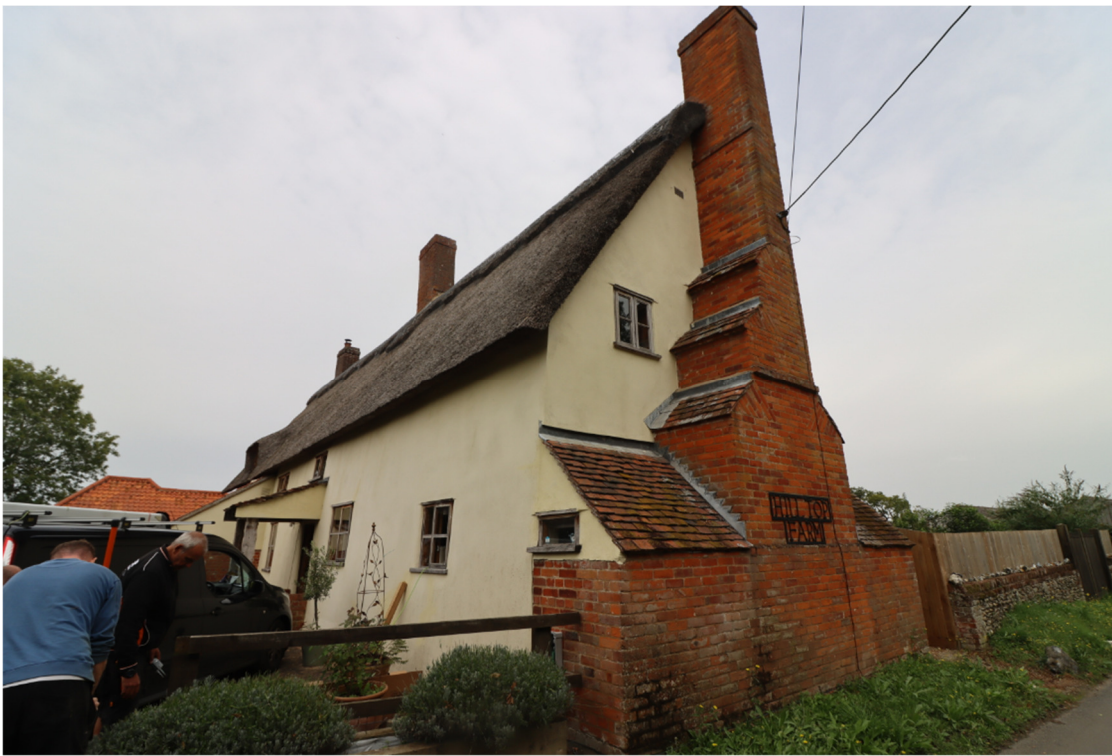
Figure 4. View from the road, looking at the Southeast gable and Southwest elevation and the former farm courtyard entrance with C20th porch added after the fire (see Figure 2 above). No change.
