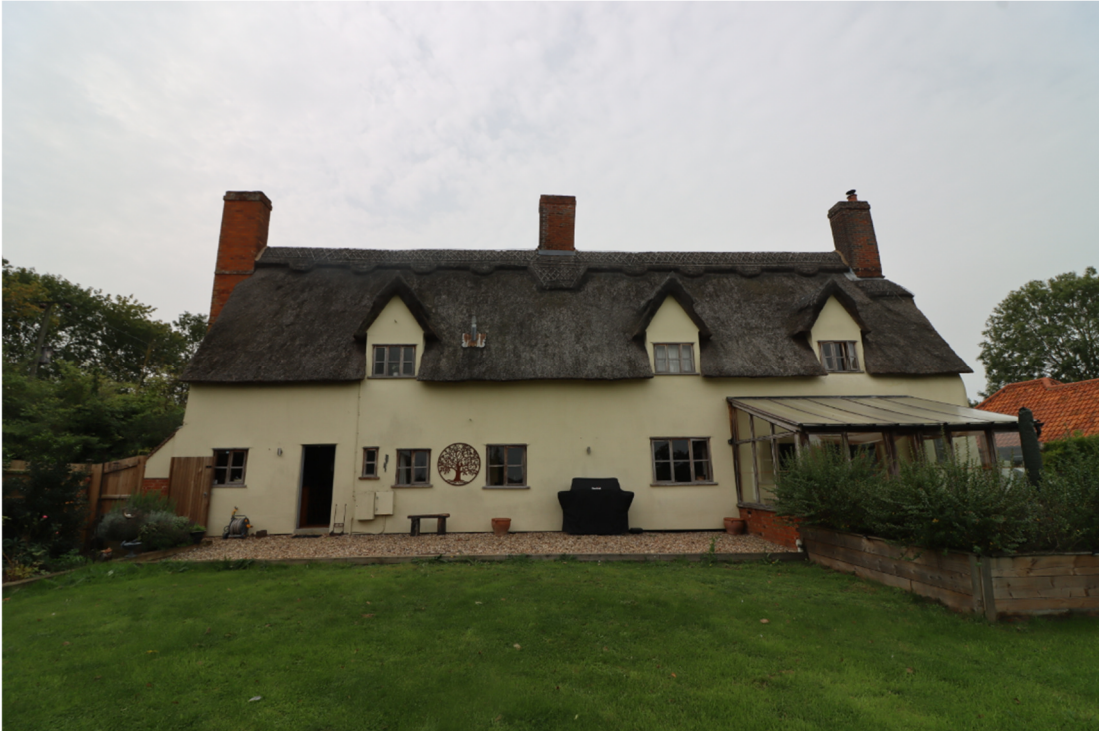
Figure 5. View of Northeast Elevation. The Sun Room is on the right.
