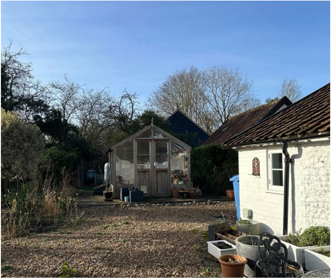
Gable of Cartlodge viewed from rear/side of Swan Cottage
