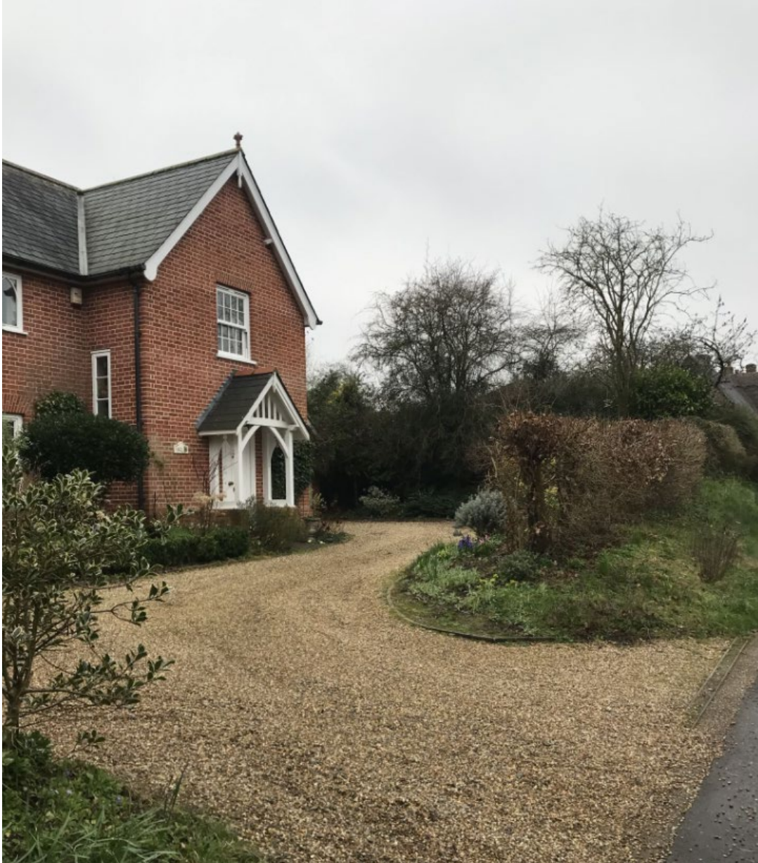
View looking towards Cartlodge from Brook Cottages
