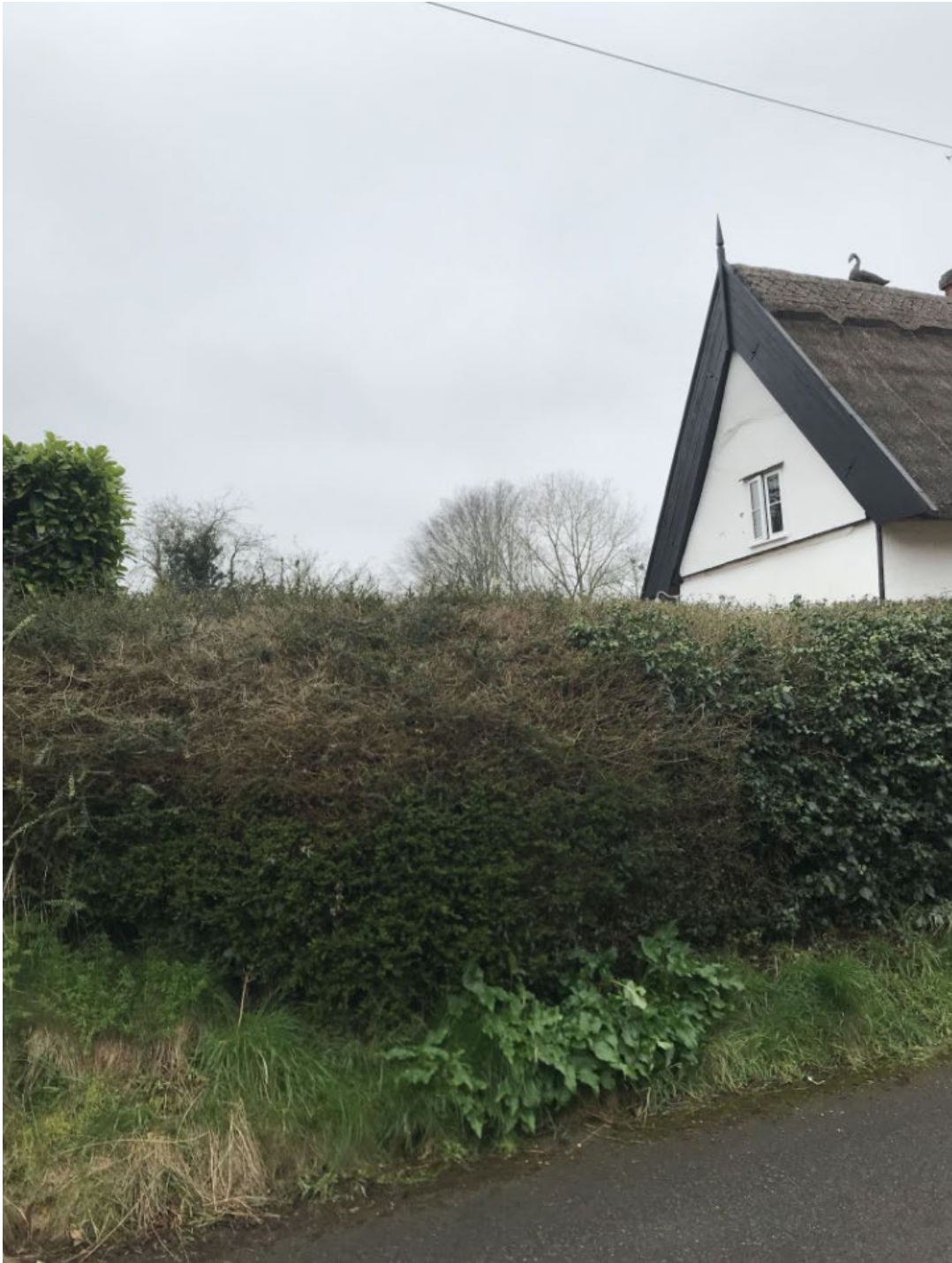
View looking towards Cartlodge from highway outside Swan Cottage
