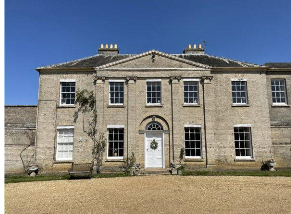
Front elevation of The Old Rectory
