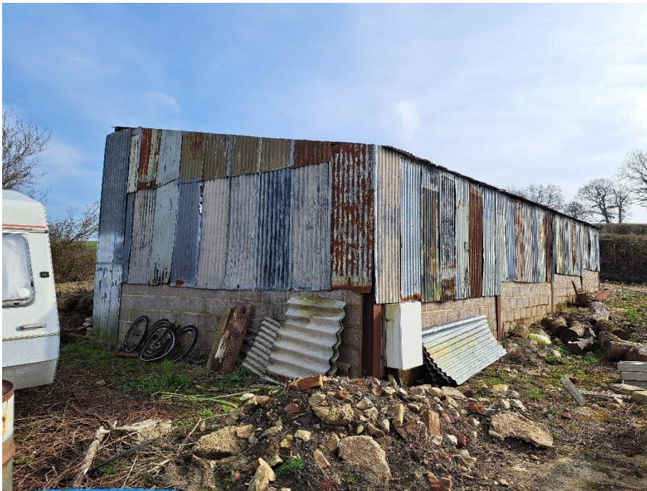
Photograph 1. Southwest and northwest elevations
