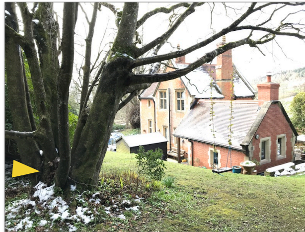
Photograph 2: Showing T2 and adjacent bank towards lodge.
