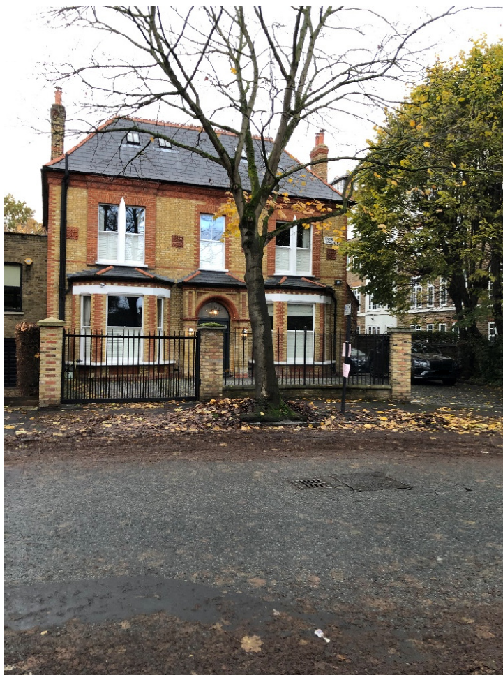
Brick piers and railings to street boundary
