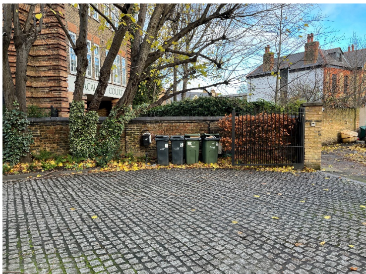
Bin store area and boundary wall
