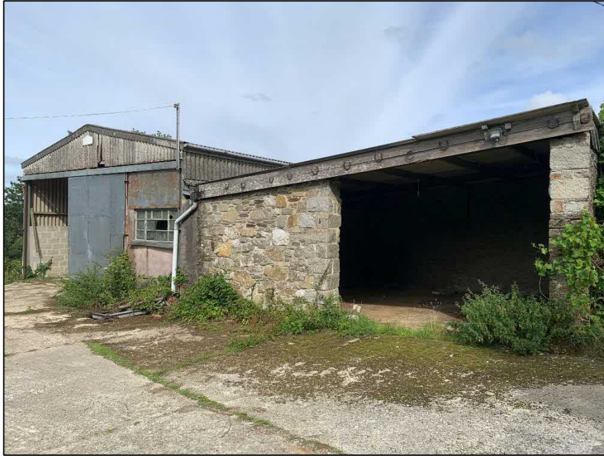
Photograph 1– View of the west aspect.
