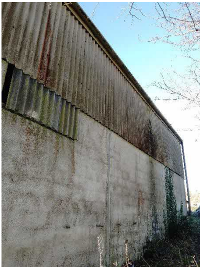
Photograph 3 – View of the north aspect.
