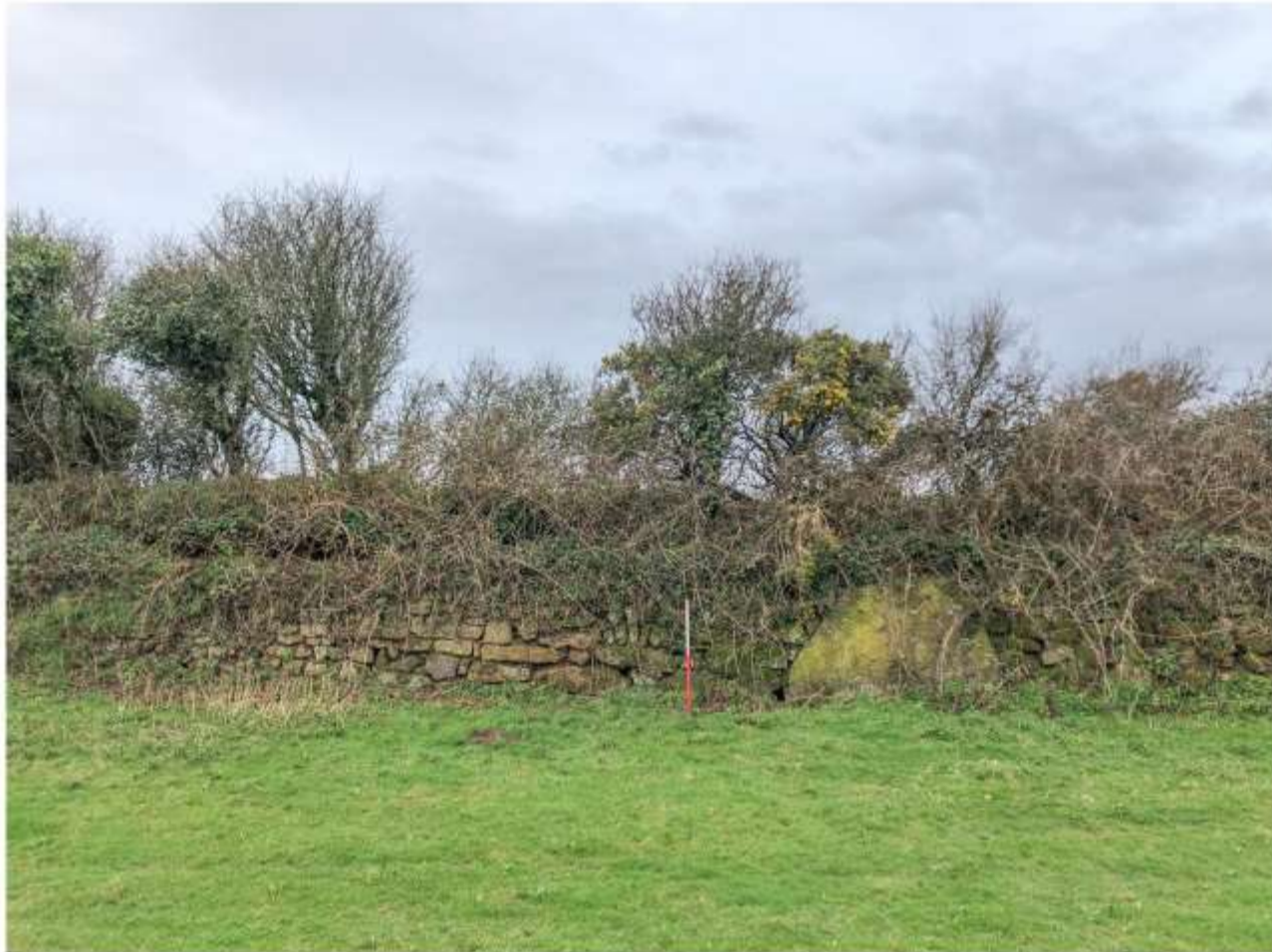
ii) east (external) face of B19 showing well coursed stone facings and the incorporation of a large earthfast boulder.
