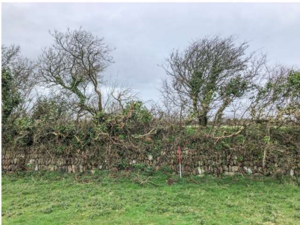
iii) B16, southern face, 1.2m high but built like the other post-medieval hedges of the walkover area of coursed regular, vertically set granite blocks.
