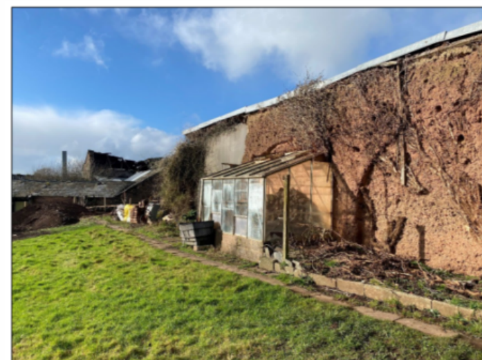
Modern lean-to greenhouse to be removed
