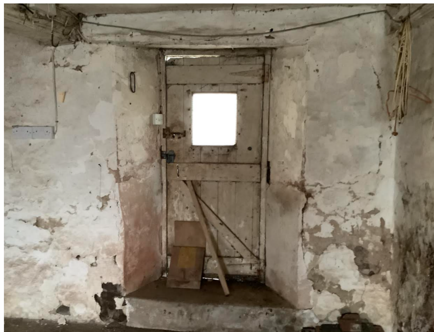
Existing Panelled Pine Door with Polycarbonate window pane.
