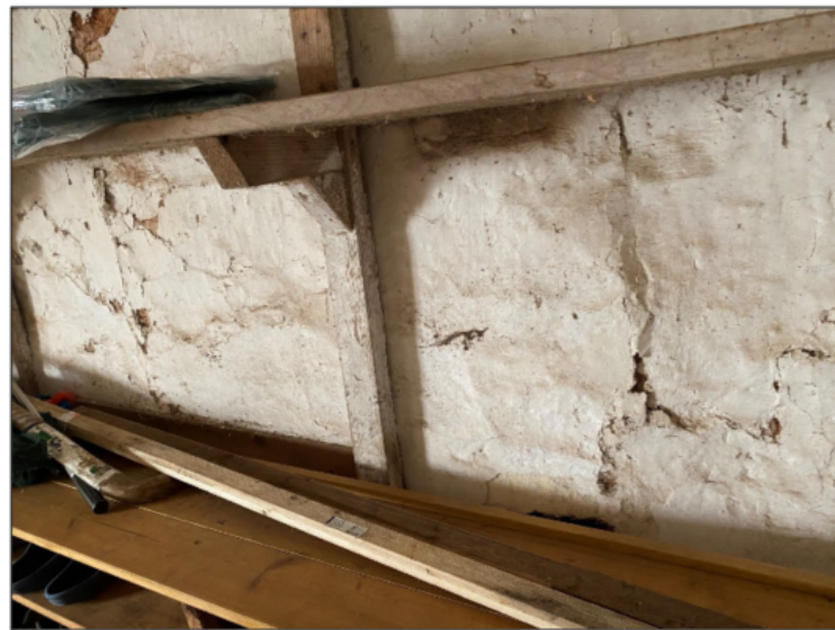
Former Doorway Outline
