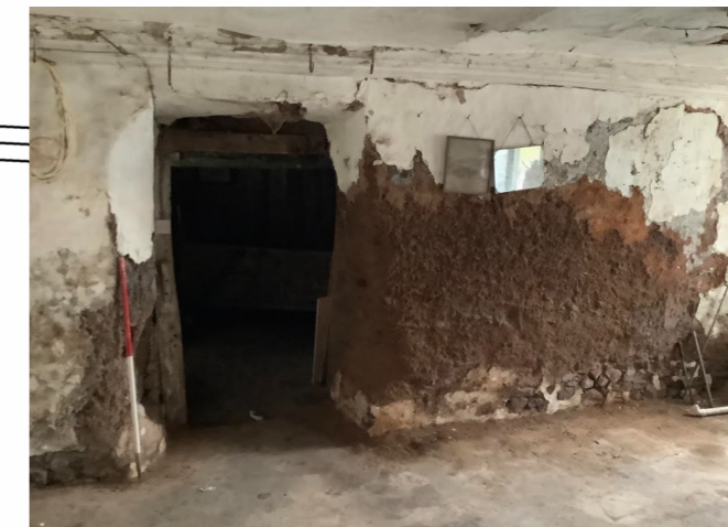
Photo showing Existing Door Oak Frame and exposed Cob Wall
