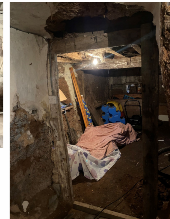
Photo showing Existing Door Oak Frame and exposed Cob Wall
