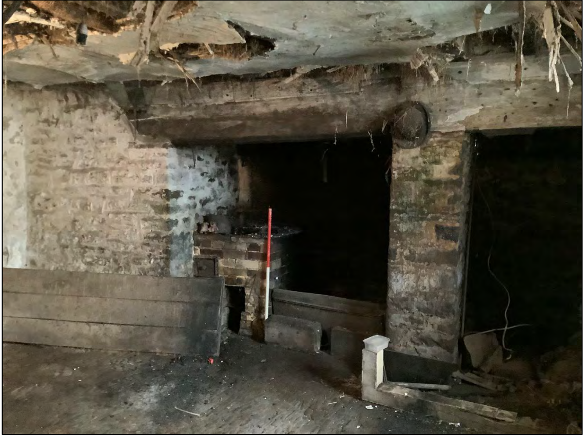
Figure 42: The large walk-in smoker hearth in the south of Room 10. A Victorian laundry wash is present within the hearth opening (left).
