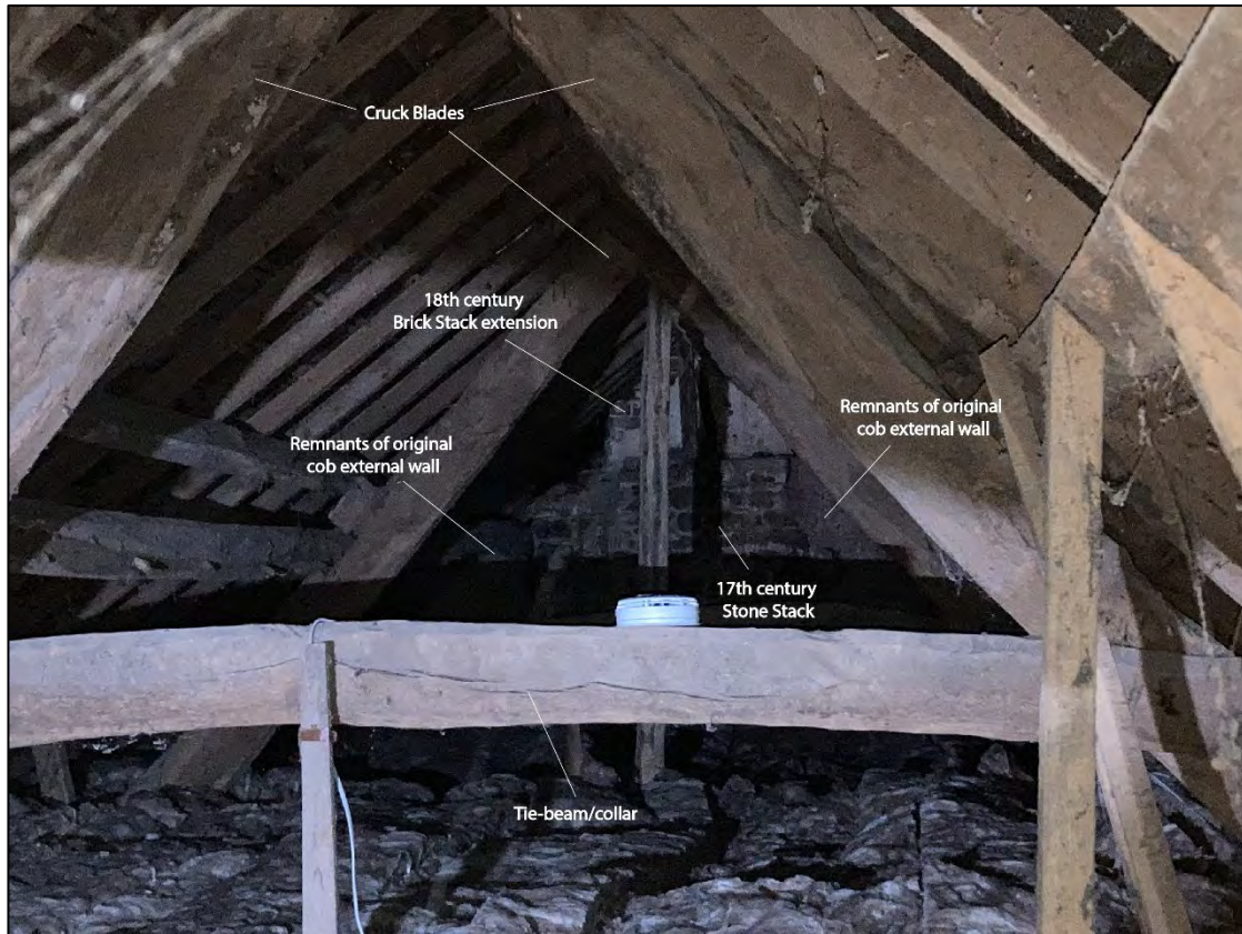
Figure 26: Hall House Roof Space. View to the eastern end.
