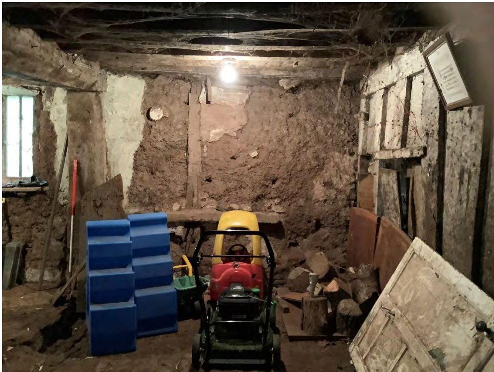
Figure 40: Possible window opening to the south of Room 9. Now filled in. Oak plank-and-muntin screen (right) separating Rooms 9 and 10.
