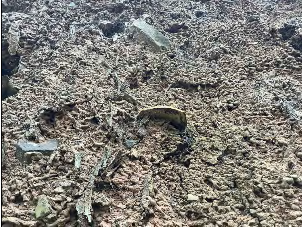
Figure 55: 18th century china pottery within the fabric of the cob wall.
