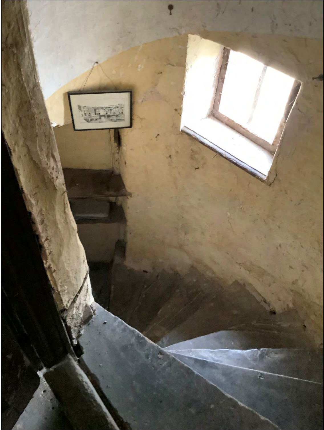
Figure 19: Likely late 16th century stairwell with oak stairs to the south west of the hall house. Built as an extension beyond the southern external rubble and cob wall to the newly installed Room 4.
