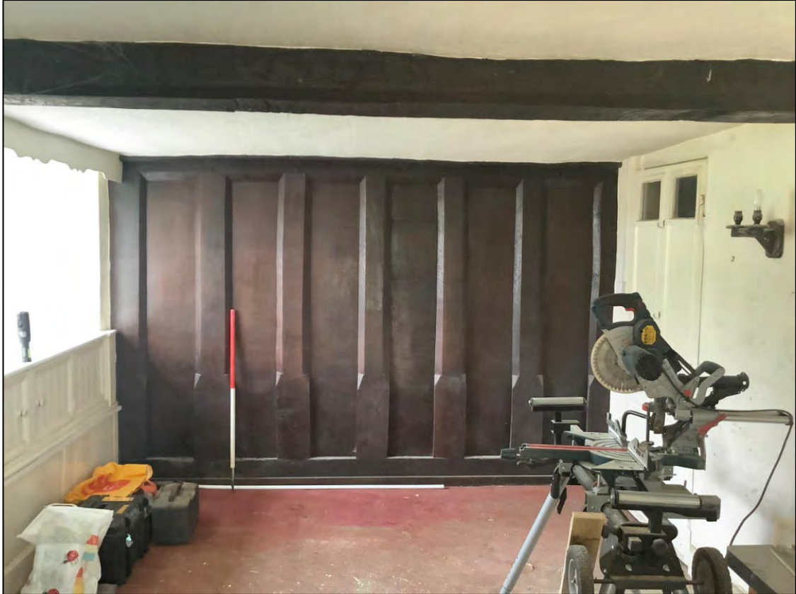
Figure 17: Oak plank-and-muntin screen separating Room 2 from Room 1, large Victorian window cavity (left) and oak crossbeam (top). There is no evidence of the original hall house superstructure beyond the west of this crossbeam suggesting that the photograph is taken from the likely 19th century extended end of the building.
