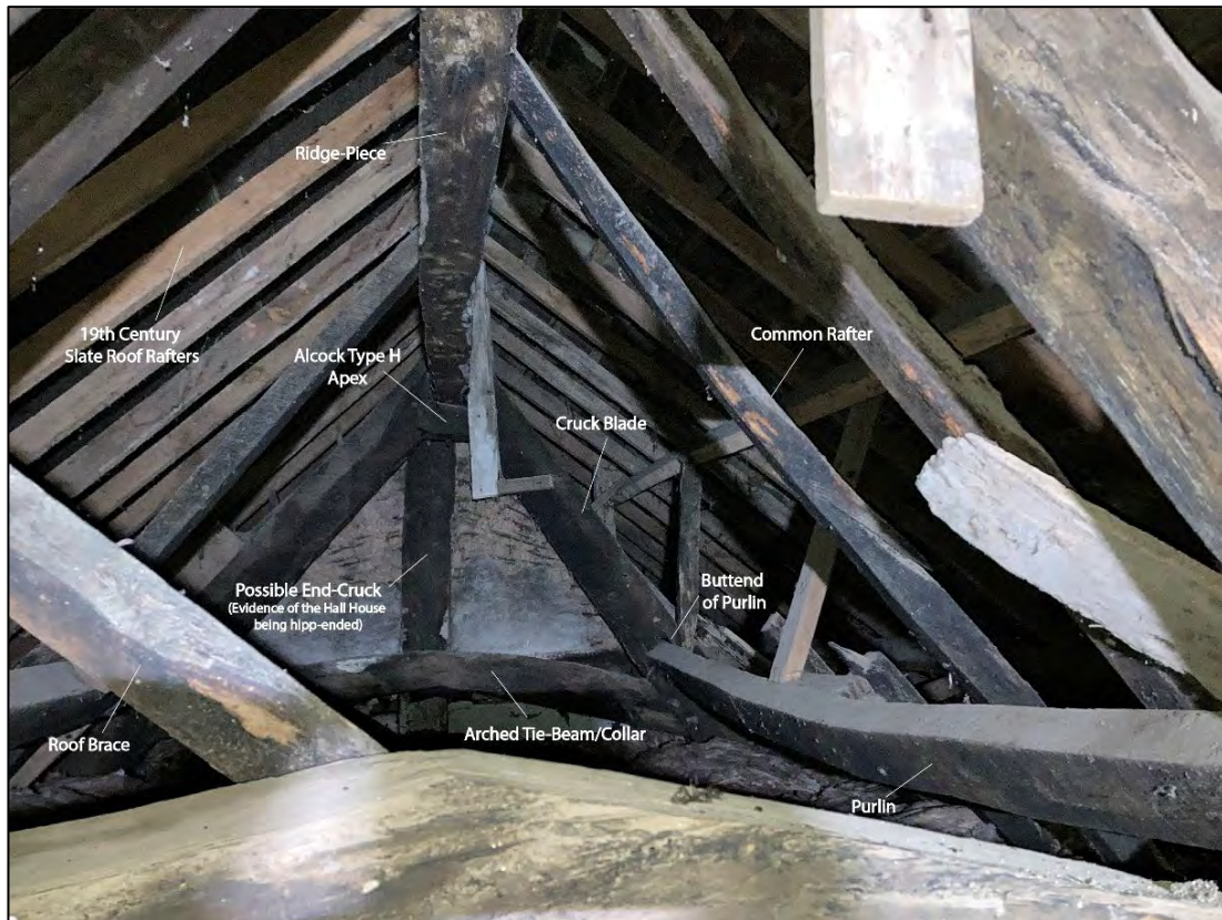
Figure 23: Hall house roof space. View to the western gable end.
