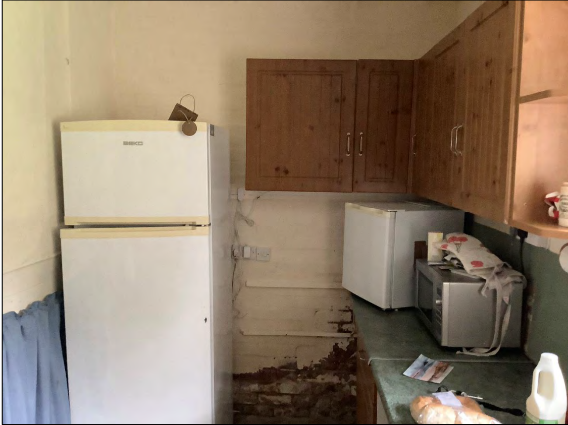
Figure 51: Brick wall between what is now the kitchen (Room 15) and Room 16.
