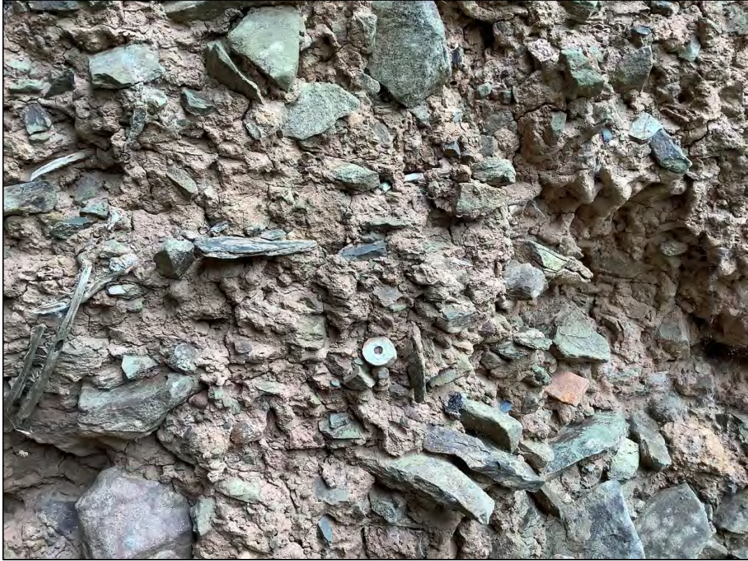
Figure 59: fragments of post-medieval tobacco pipe within the eastern cob walls fabric.
