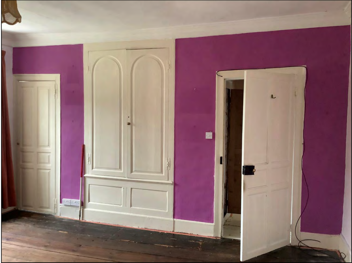
Figure 50: Late 17th century cupboard (centre) and power room (left) within Room 17.
