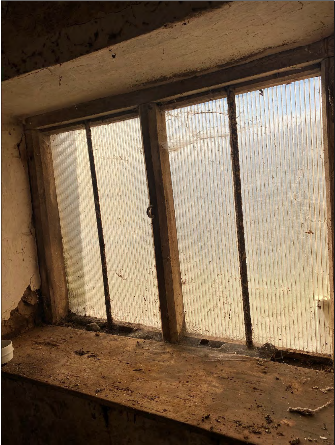
Figure 63: Historic window frame and ledge in Room 8 to be left in-situ, polycarbonate pane to be replaced with 12mm double glazing to provide warmth to the room and create a liveable space (Fig. 1, 3d)
