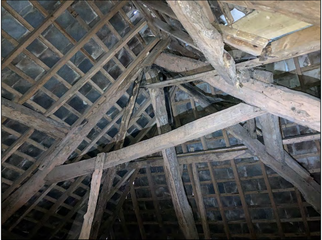
Figure 52: The hip-ended roof of the northern wing.
