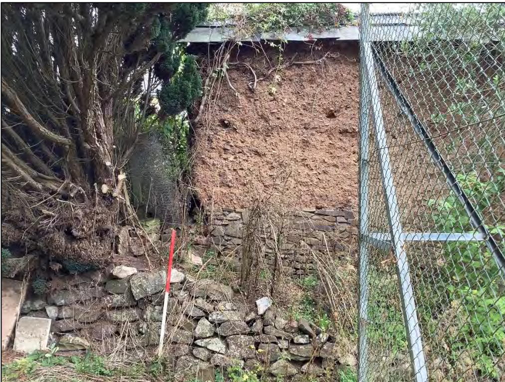
Figure 58: Cob wall to demarcating the eastern boundaries of Poole Barton.
