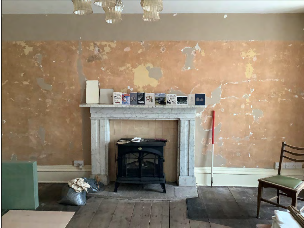
Figure 49: The marble fire surround in Room 14.
