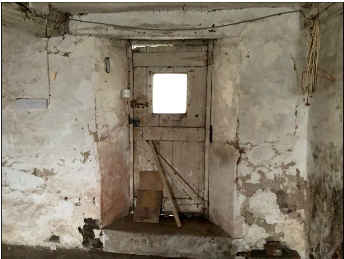
Figure 35: Room 8's doorway to the east.
