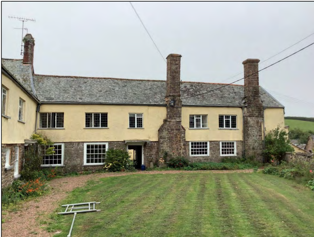
Figure 7: North elevation of the east to west axis main block demonstrating the construction of exposed volcanic rubble wall to the first floor, plastered cob above, three chimney stacks and 19th century slate roof tiles. View to the south.
