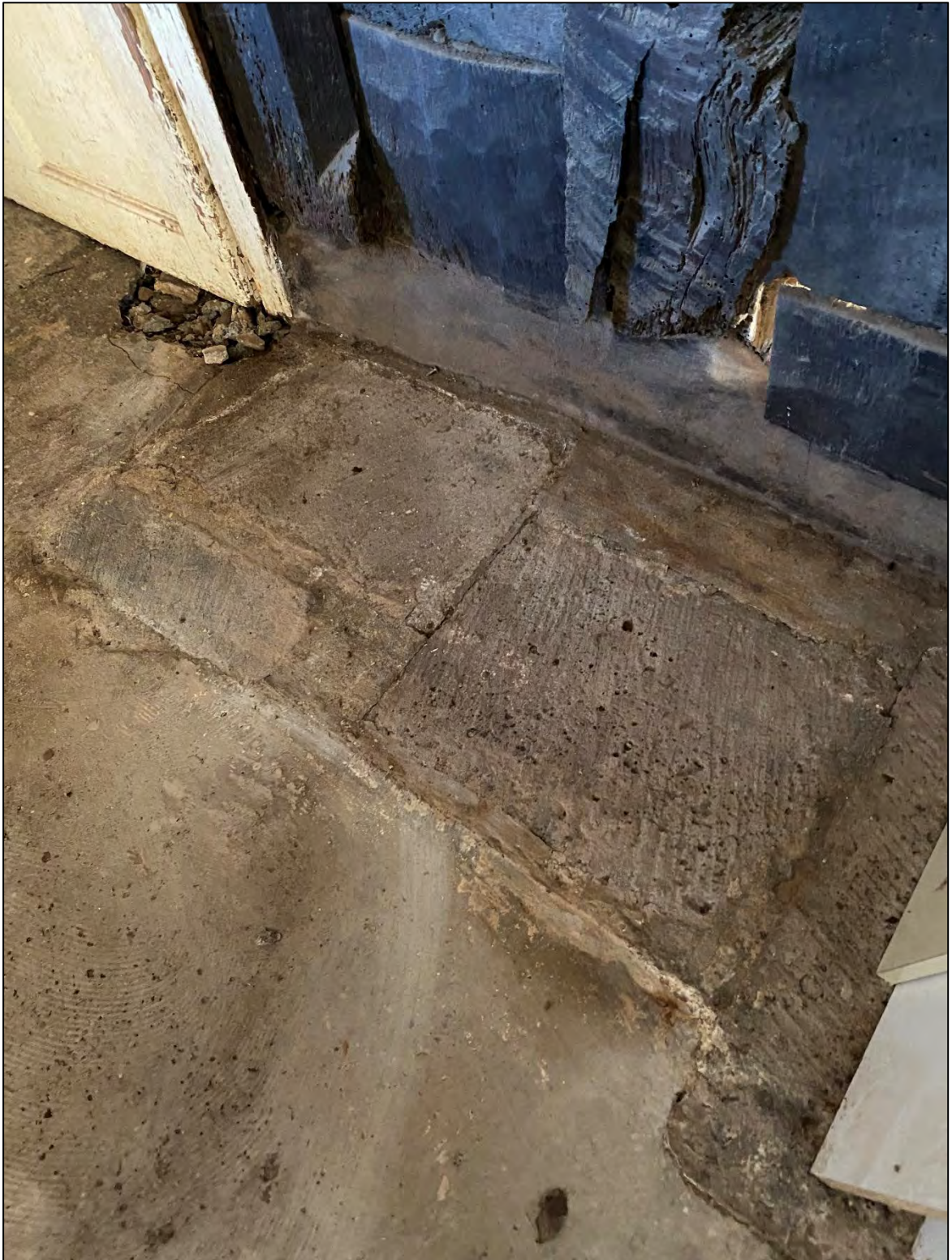
Figure 62: Historic volcanic flagstones in the south west corner of Room 1
