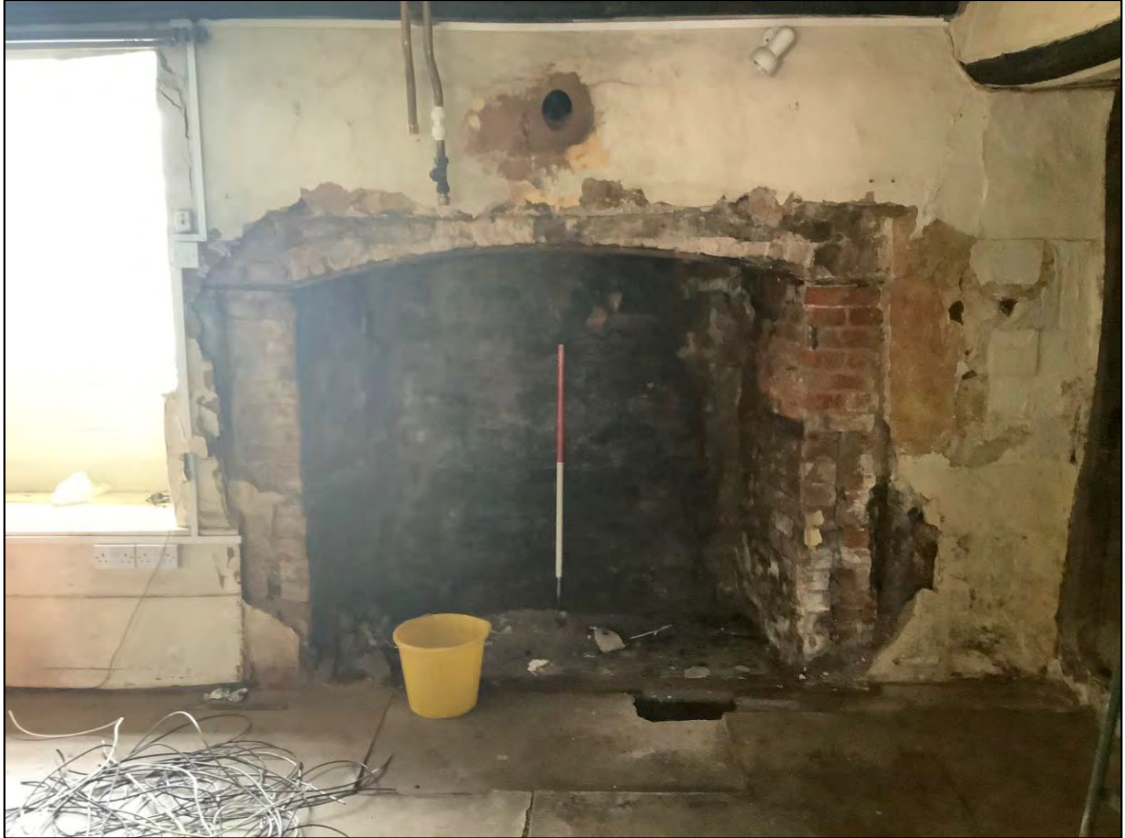
Figure 12: Brick-and-mortar lined fireplace cavity with arched brick lintel and cast-iron former.
