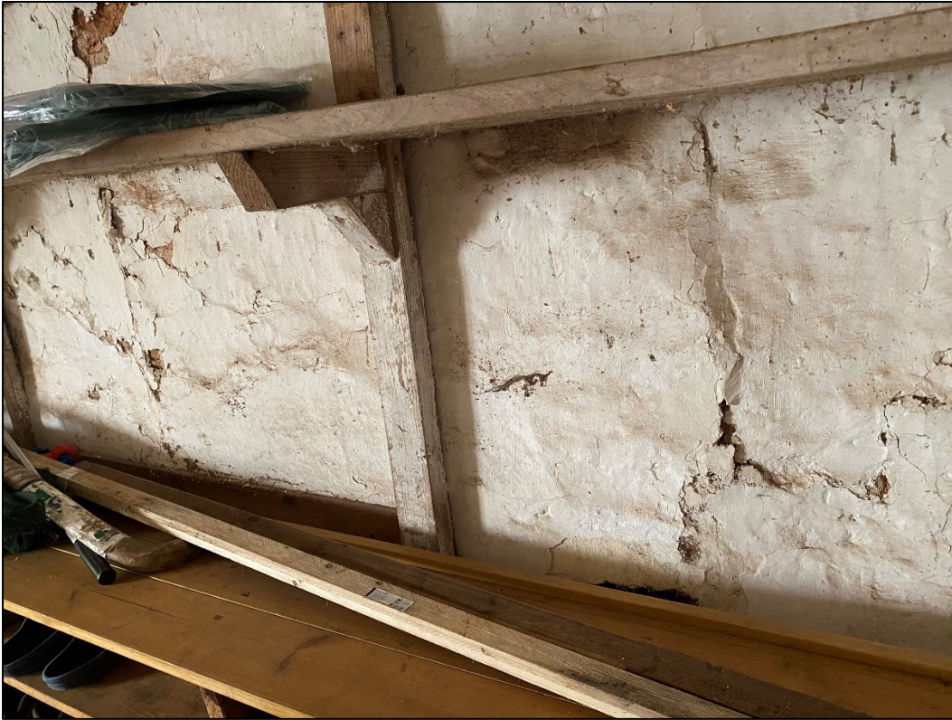
Photo 5: Former doorway outline to be reinstated between Rooms 8 and 3 (Fig. 1, 3a)
