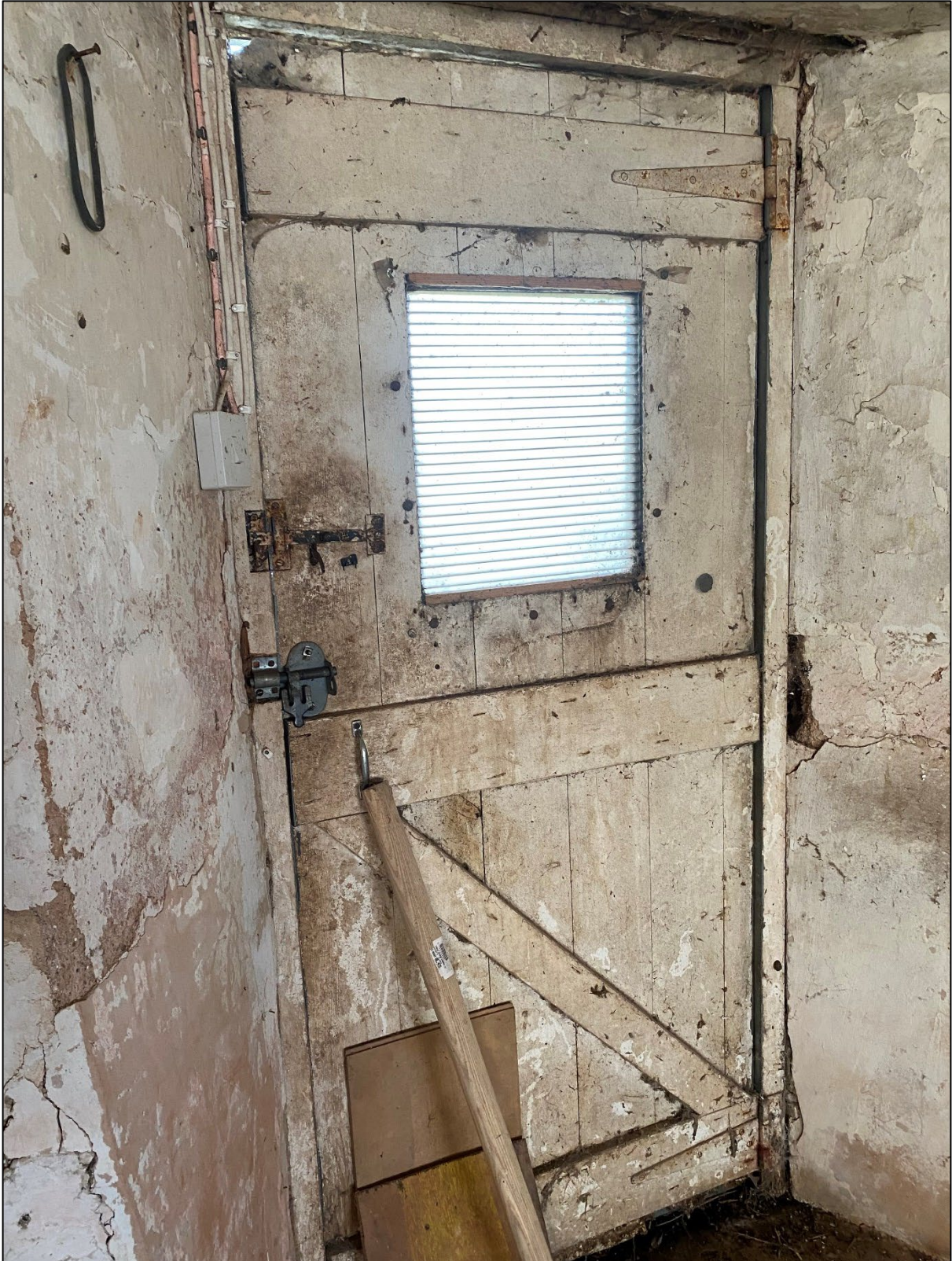
Photo 7: Pine door to be replaced with oak door of the same type on the eastern side of Room 8 (Fig. 1, 3b)
