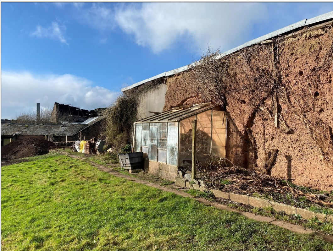
Photo 12: Modern lean-to greenhouse to be removed along the route of a curtilage cob wall (formally walled garden) (Fig. 1, 4b)
