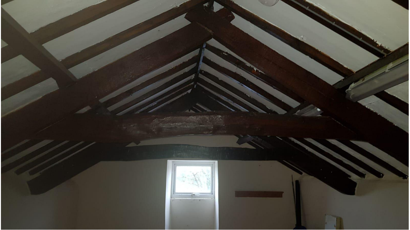
Above: Raised collar scissor trusses
