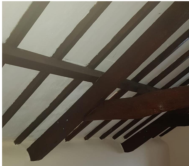
Above: Timber rafters on purlins on trusses
