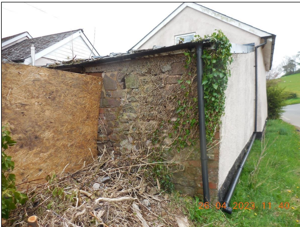
Photo 2: Northern aspect of barn with brick wall
