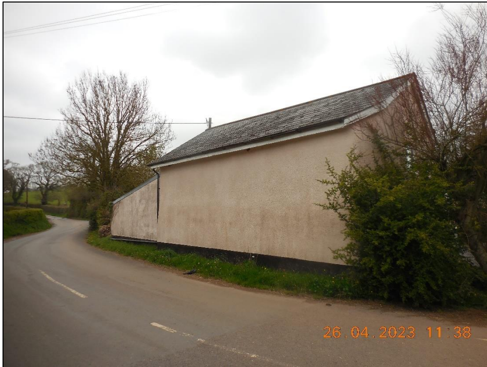
Photo 3: showing western aspect of site, hedgerow with trees in background.
