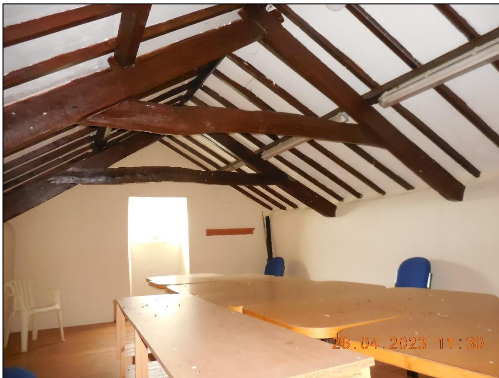
Photo 4: Interior of converted roof space of barn
