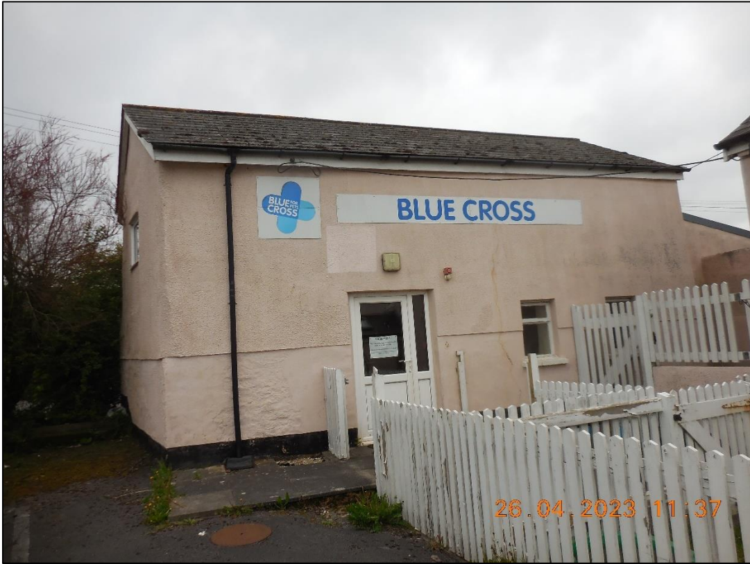
Photo 1: Exterior of eastern and southern aspect of the barn
