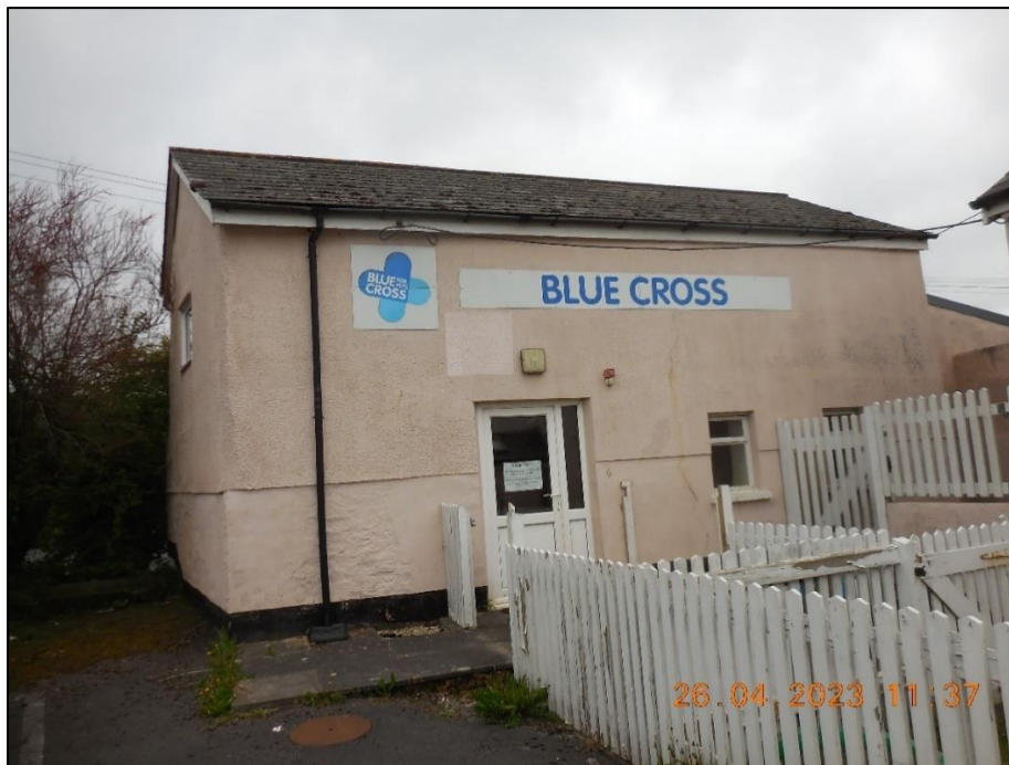
Photo 1: Exterior of barn/ shop.
