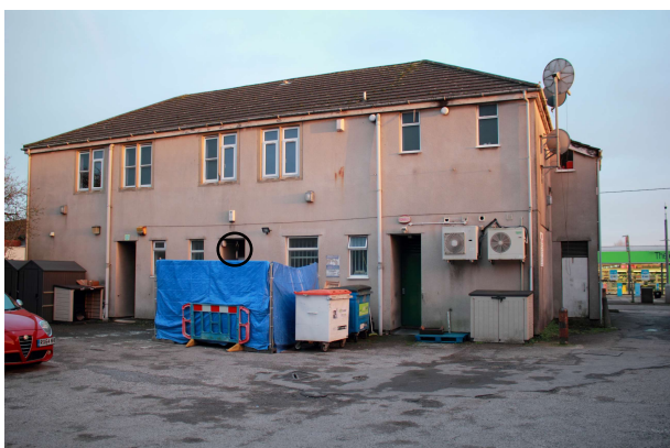
Looking south east towards Location 2
