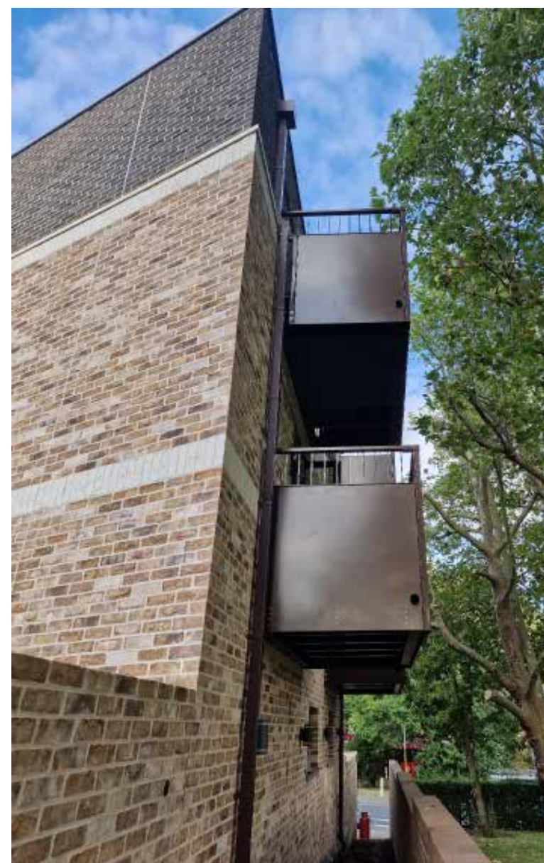
North elevation side view
