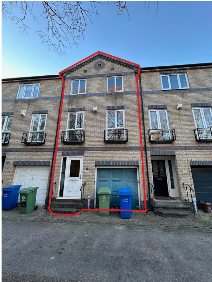
Front elevation. The existing timber framed windows are in poor condition and will be replaced, with white framed double glazed aluminium units. The metal garage door is visually dominant in the elevation.
