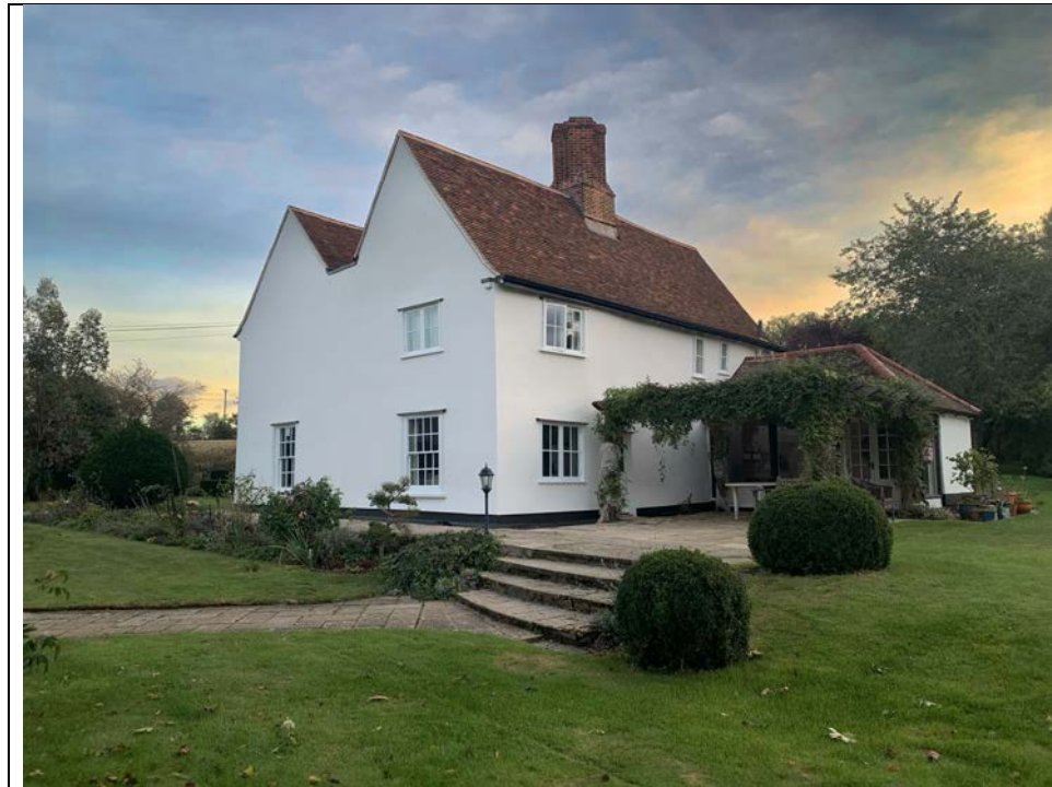
The existing Burnthouse Farm from the garden looking north east.
