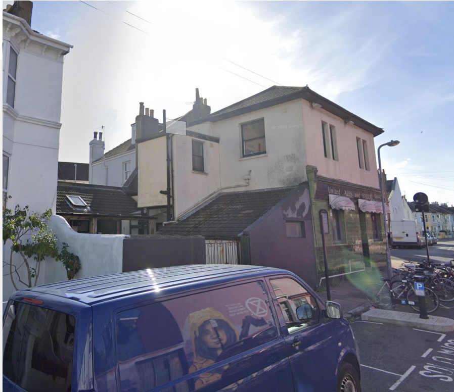
Current view from Montreal Road
