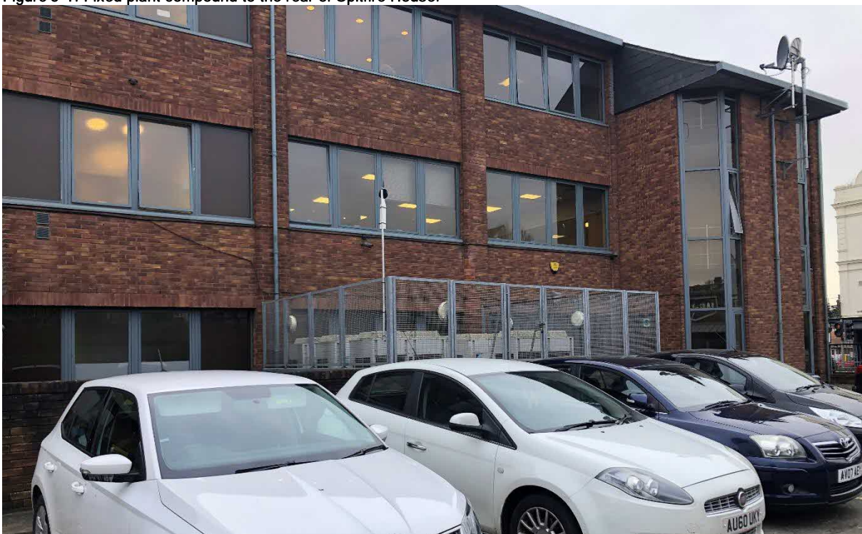
Figure 5-1: Fixed plant compound to the rear of Spitfire House.
