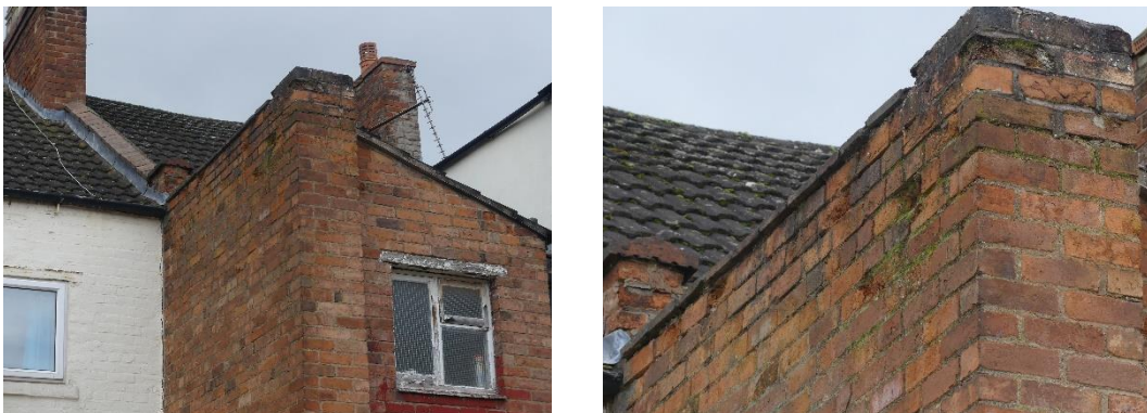
Figs. 5 & 6 Ridge, roof tiles and parapet to rear
