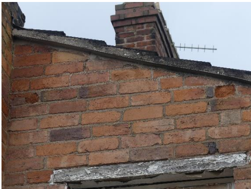
Figs. 9 & 10 Verge fully pointed (L) and bathroom window (R)
