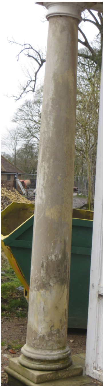
EXISTING COLUMN ON SIDE OF MAIN HOUSE
