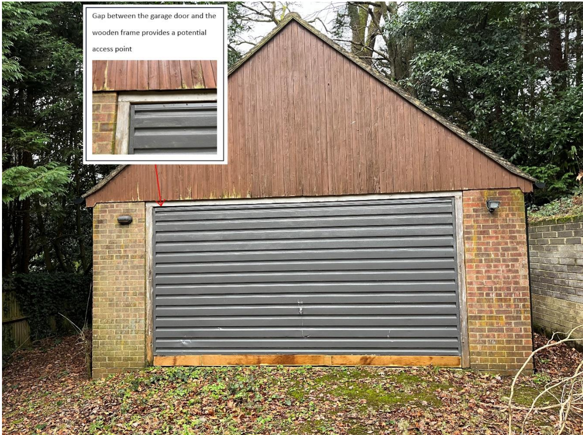
Image 4.3.1.3. Location of potential bat access points on the east elevation of the garage.
