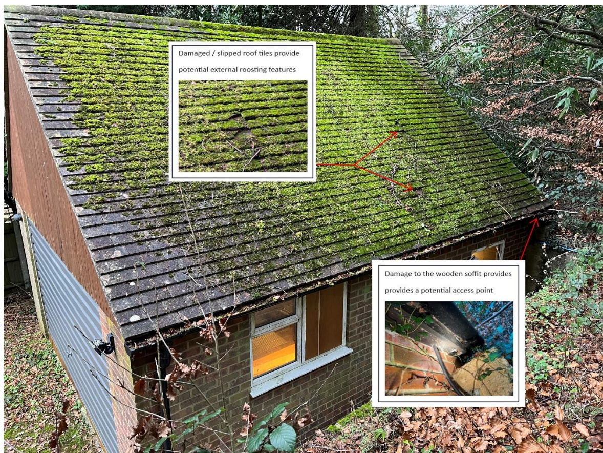
Image 4.3.1.1. Location of potential bat access points and potential external roost locations on the north elevation of the garage.
