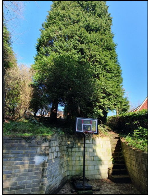
Fig 2: Group #04 atop retaining wall
