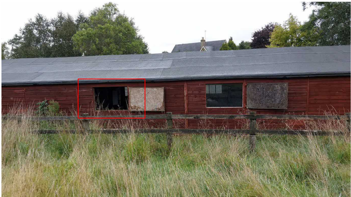
Plate 4: Image showing the missing windowpane (red shape) at the west elevation of the stables.
