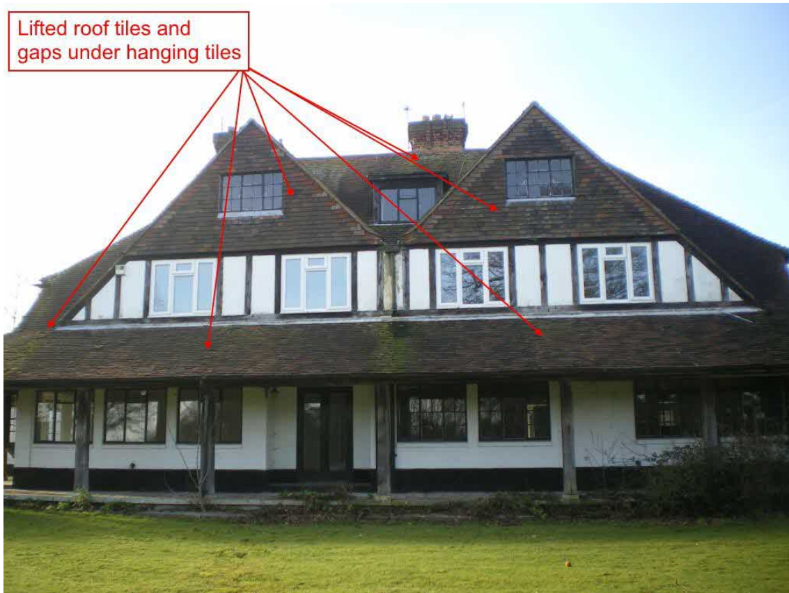
Image 4.3.1.2. Location of potential bat access points and potential exterior roof features on the east elevation of the house.
