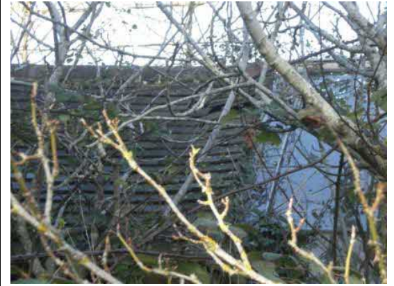
Under roof tiles
