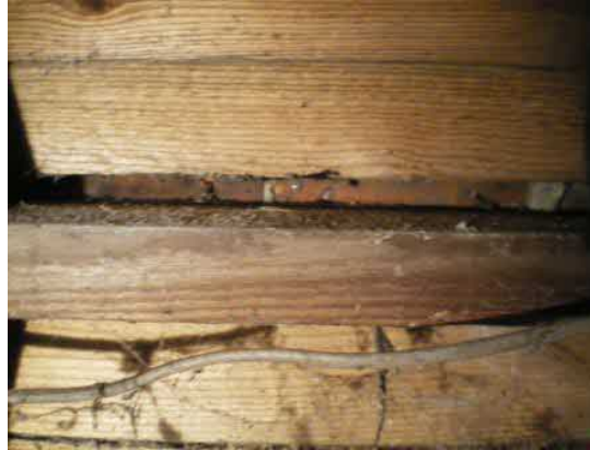
Under wooden cladding and sarking boards
