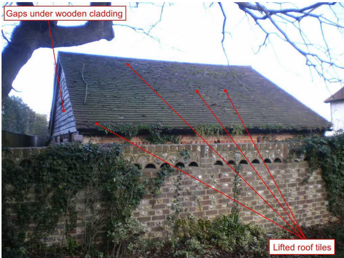
Image 4.3.1.6. Location of potential bat access points and potential exterior roof features on the south and west elevations of the garage.
