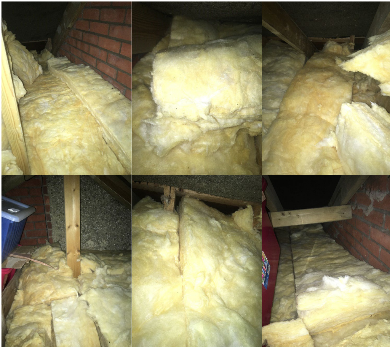
Image set 3. Inside of roof space
